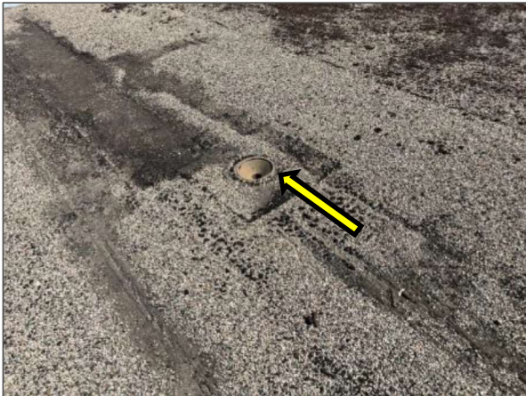
Missing debris strainers were noted atop Roof Section 6.
