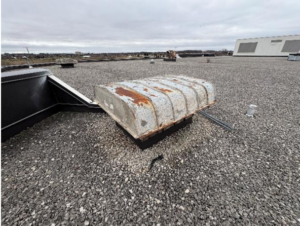
Figure 5: Exhaust hoods are typically corroded.
