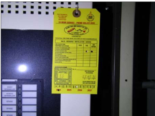
The fire alarm system was observed to be past-due its annual inspection date.
