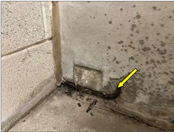
View of the area of exposed rebar noted in the southeast portion of the first floor.
