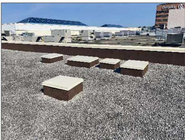
View of redundant HVAC curbs noted in the north portion of the primary IRMA system.
