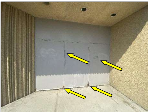
View of typical worn corrosion and worn finishes noted on hollow metal doors on the east elevation of the Site Building.
