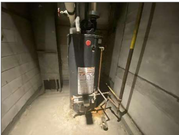
View of the "Rheem" natural gas-fired DHW heater.
