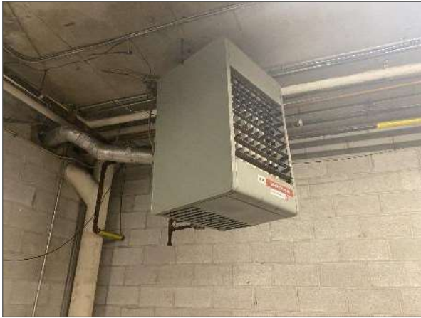
View of a typical suspended unit heater.
