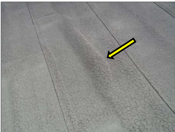
Areas of membrane blistering of the modified bitumen membrane roof system were noted atop Roof Section A3 in multiple locations.
