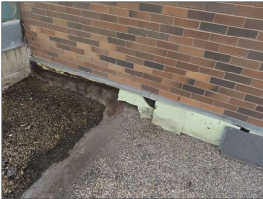
View of an area of missing insulation and lack of flashing atop Section 9 of the Site Building.
