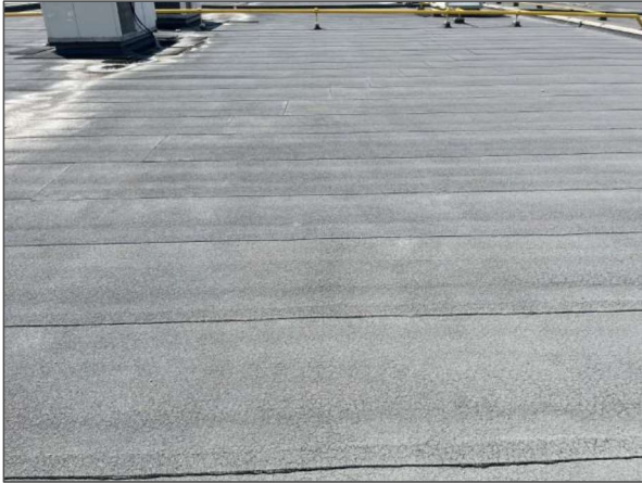
General view of a typical modified bitumen membrane Roof Section A4 serving the Site Building.
