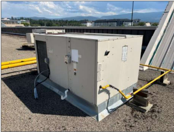
General view of a typical rooftop packaged HVAC unit.
