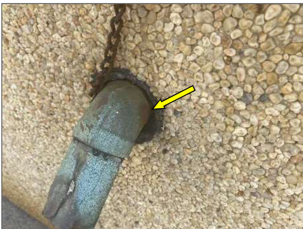
View of a typical unsealed penetration noted on the south elevation of the Site Building.
