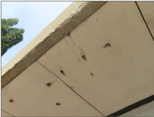
View of damaged and cracked soffit on the south elevation the Site Building.
