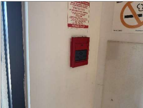
View of a typical manual pull station.
