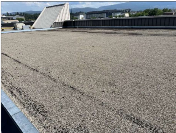
General view of the BUR membrane serving Roof Section A6.
