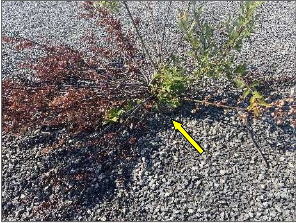
View of a partially obstructed roof drain noted in the central portion of the primary IRMA system.
