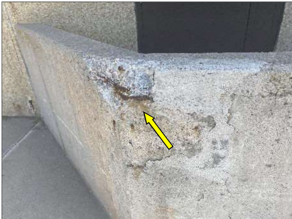
View of an area of deteriorated concrete noted at the concrete stairs at the southeast portion.
