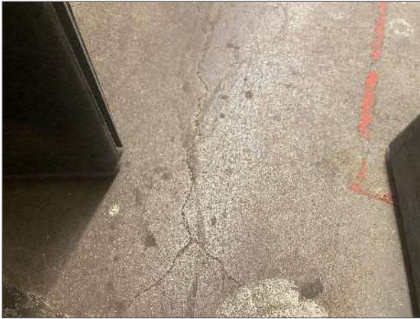
View of typical cracking in the exposed concrete floor slab noted within the shipping/receiving area.
