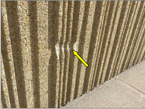
View of deterioration in the precast concrete wall panels noted on the south elevation of the Site Building.
