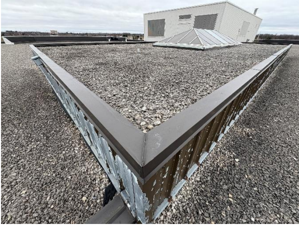
Figure 9: Peeling paint finish at metal siding.
