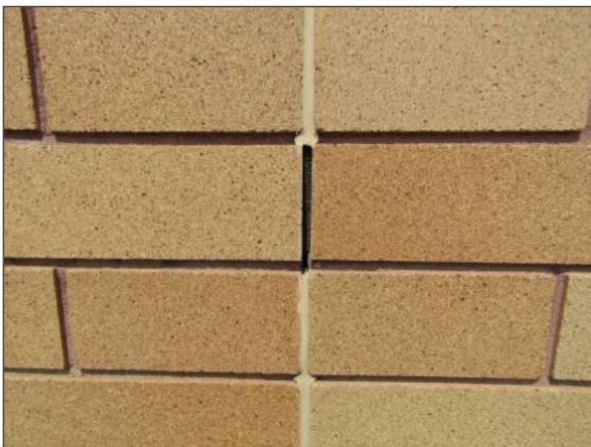
Missing transition sealant were noted on the south elevation.
