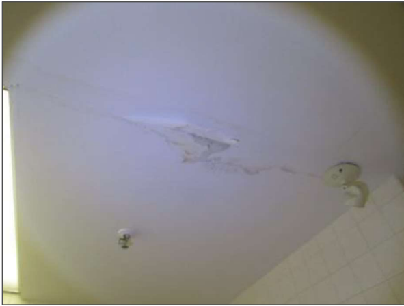
Moisture damage/stained gypsum ceiling board was noted in multiple locations of the Site Building.
