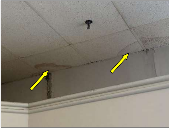
View of moisture/water-stained ceiling tiles noted adjacent to the south entrance of the Site Building.
