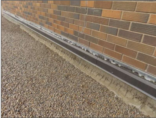
View of typical deteriorated membrane edge atop Sections 8 and 9 of the Site Building.
