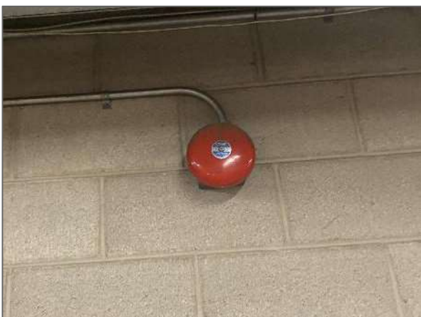
View of a typical alarm notification appliance (i.e., a fire bell).
