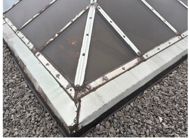
Figure 10: Deteriorated face sealant observed at skylight.
