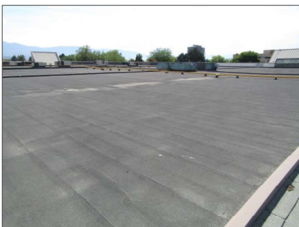
General view of a typical modified bitumen membrane Roof Section A3 serving the Site Building.
