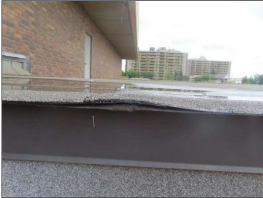
View of unadhered modified modified membrane atop raised modified bitumen membrane roof system atop Section 9 of the Site Building.
