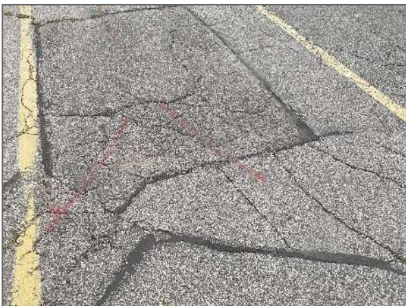
View of typical deteriorated asphalt pavement noted to the south of the Site Building.
