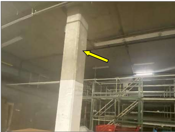
View of a typical reinforced concrete column and capital supporting a concrete floor slab in the southeast portion of the Site Building.
