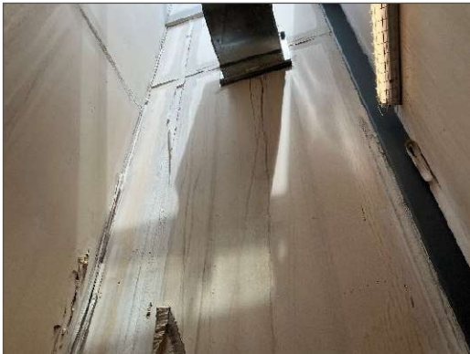
View of moisture staining noted at the gypsum board below the decorative glass exterior feature at the southwest corner of the Site Building.
