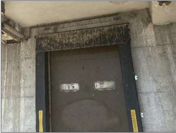
View of a typical aged sectional metal overhead door.
