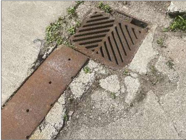
View of deterioration in the cast-in-place concrete apron serving the shipping/receiving area.
