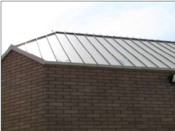
General view of a typical sloped Metal mansard style roof area serving the Site Building.
