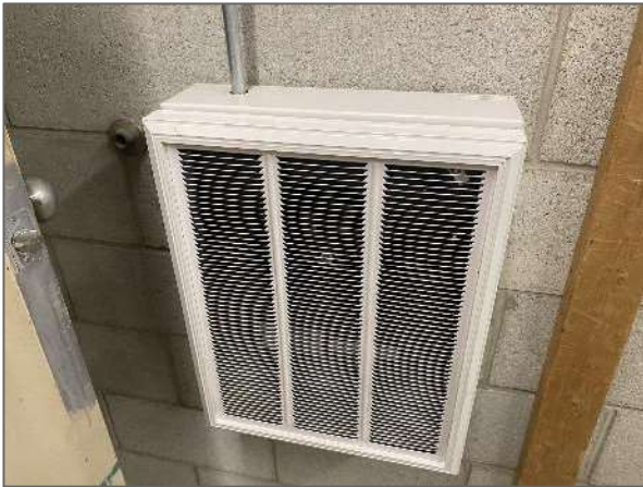
View of a typical electrically-powered wall-mounted forced air heater.
