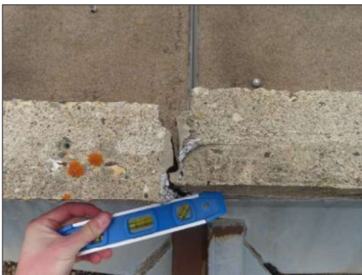
View of typical minor movement noted on precast concrete panels on multiple elevations the Site Building.
