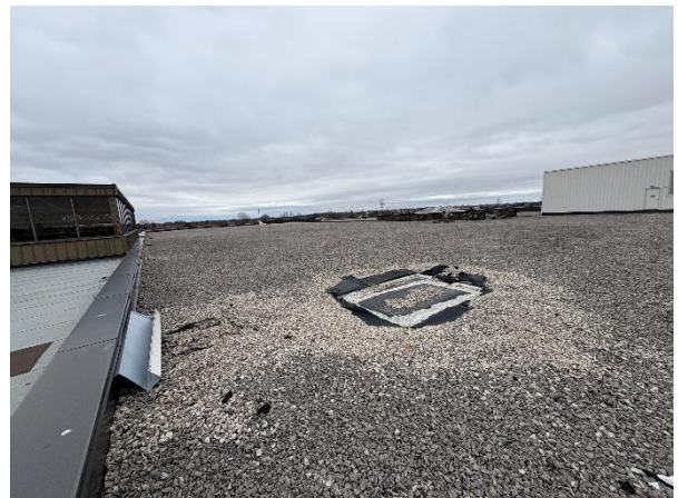
Figure 8: Damaged metal panel and flashing are visible on the west wall of the roof.
