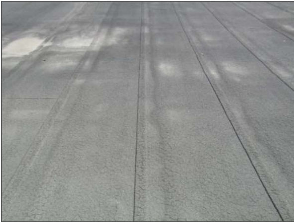
Areas of membrane crazing of the modified bitumen membrane roof system were noted atop Roof Section A4 in multiple locations.
