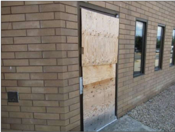
A damaged SG door was noted on the north elevation.
