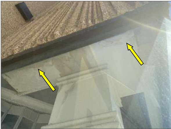
View of water damage in the gypsum wall and ceilings boards, reportedly due to a previous pipe leak noted adjacent to the south entrance of the Site Building.
