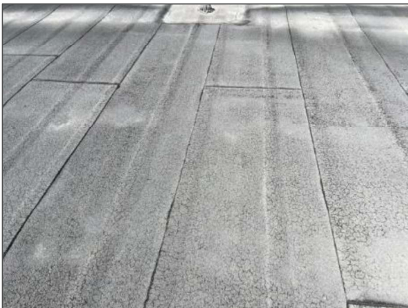
Areas of membrane crazing of the modified bitumen membrane roof system were noted atop Roof Section A5 in multiple locations.
