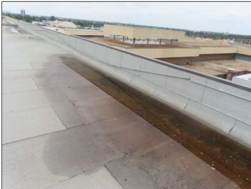
View of typical evidence of ponding atop multiple sections the Site Building.
