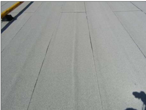
Areas of membrane wrinkling of the modified bitumen membrane roof system were noted atop Roof Section A1.
