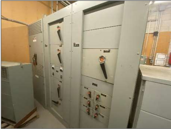
View of the "Federal Pioneer" main electrical disconnect switch.
