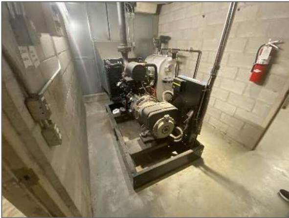
View of the "SDMO" diesel-fired emergency generator.
