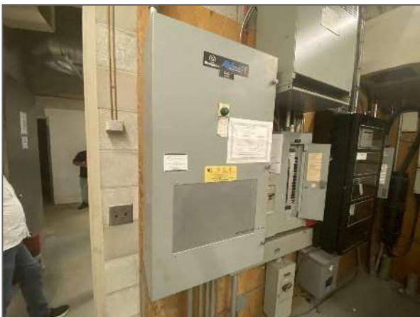
View of the "Westinghouse" automatic transfer switch.
