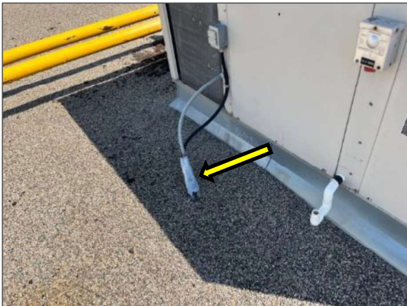
Poorly executed service penetrations were noted in multiple locations atop the Roof Sections of the Site Building.
