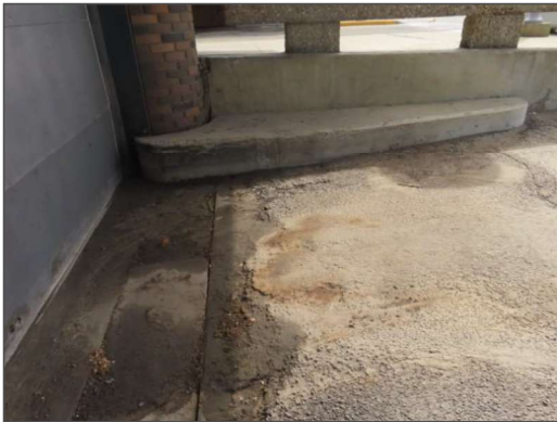
View of deteriorated asphalt surfaces adjacent to the south elevation of the Site Building.
