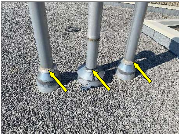
View of deteriorated sealants noted on vent penetrations in the southeast portion.
