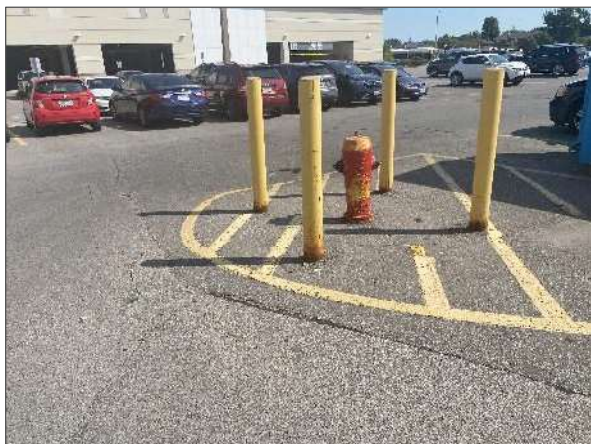
View of a typical private fire hydrant located to the east of the Site Building.
