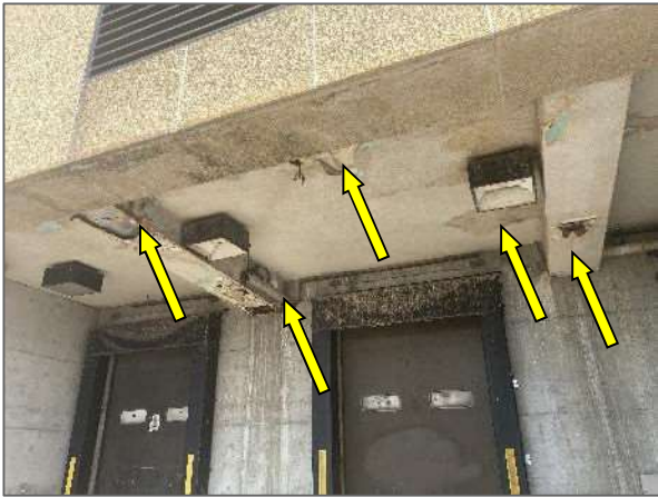
View of water-damaged gypsum board and exterior finishes on the soffit above the shipping/receiving area.
