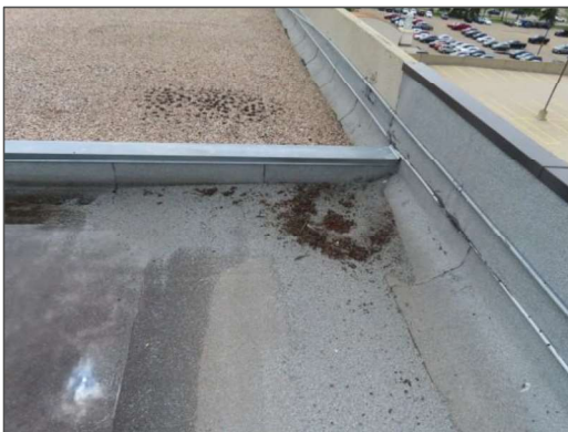
View of typical degranulation and deterioration of the modified bitumen membrane atop multiple sections of the Site Building.
