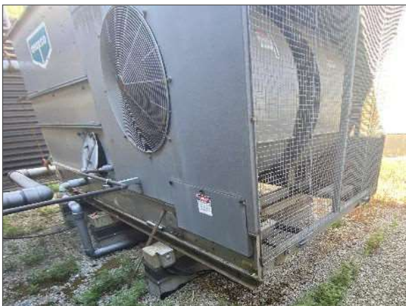
View of the "Evapco" cooling tower.
