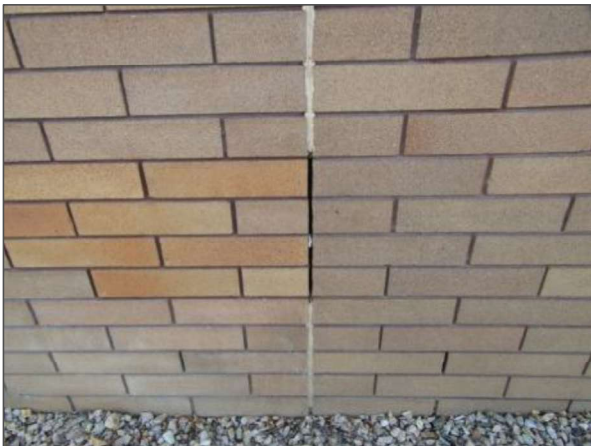
Missing transition sealant were noted on the north elevation.
