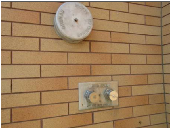
General view of the FDC noted on the south elevation.
