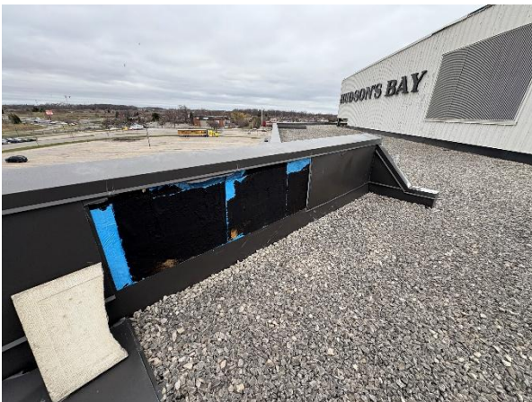
Figure 7: Missing parapet cladding removed, exposed membrane flashing.
