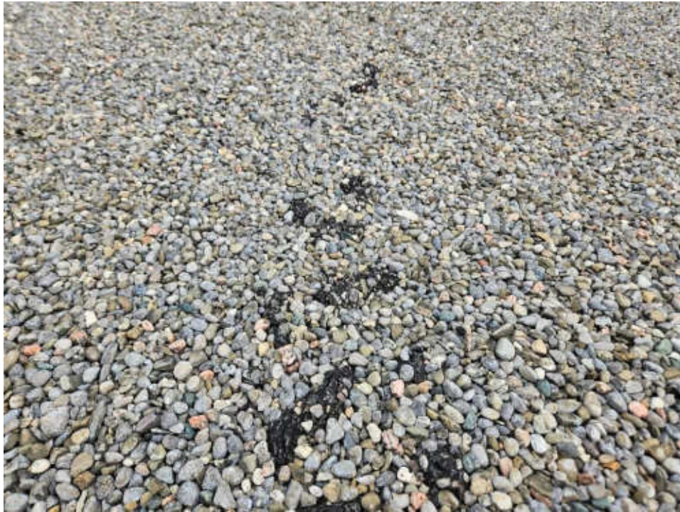
Photo #13: Asphaltic Bleed-out at Main BUR Roof
