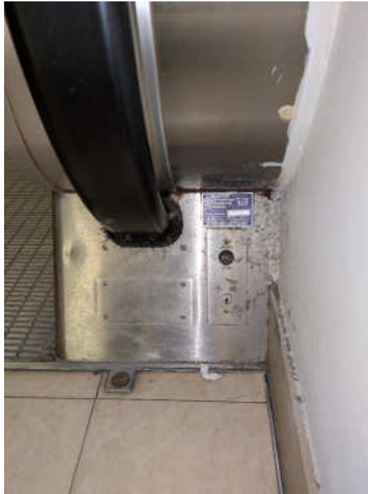
Photo #13: Escalators Handrail Inlet
