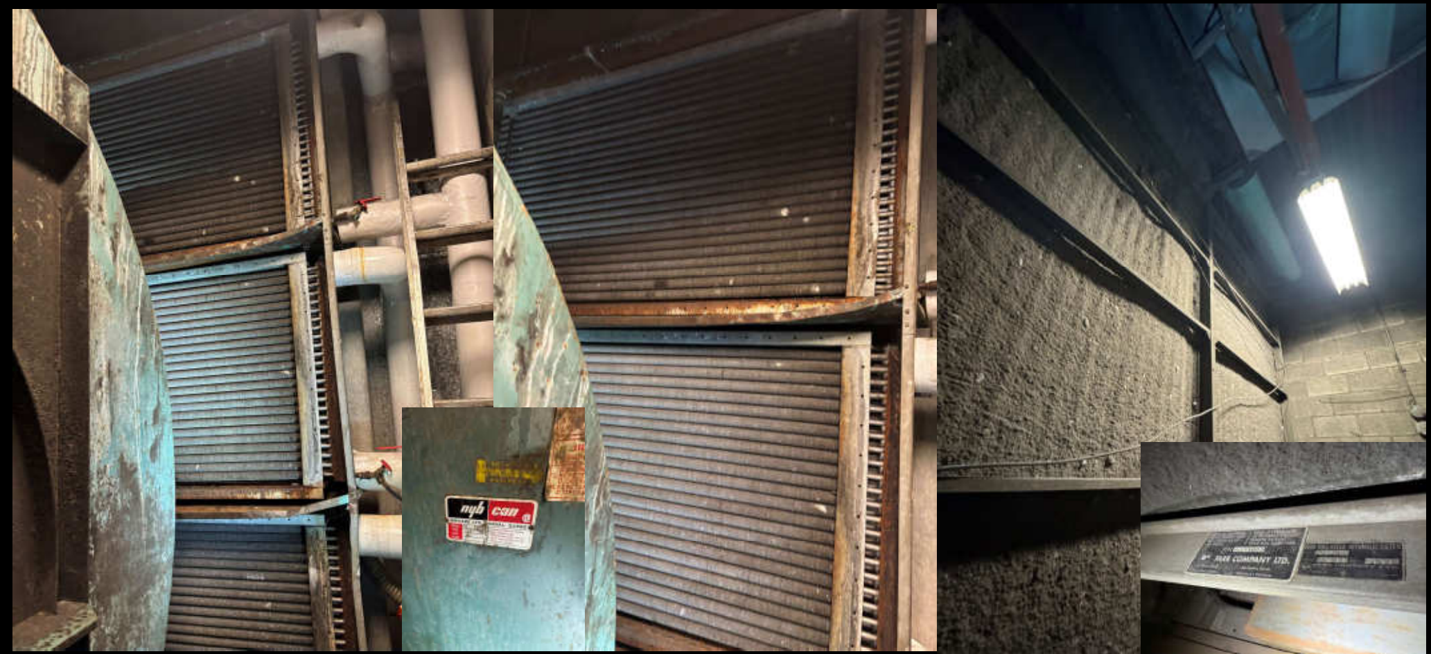
Condition of HVAC System - Central Air Handling supply equipment has not been service in a long time. Note the thick layer of dirt and debris on the air filter media
