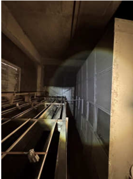
Photo #15: AHU-1 Mixing Air Plenum
