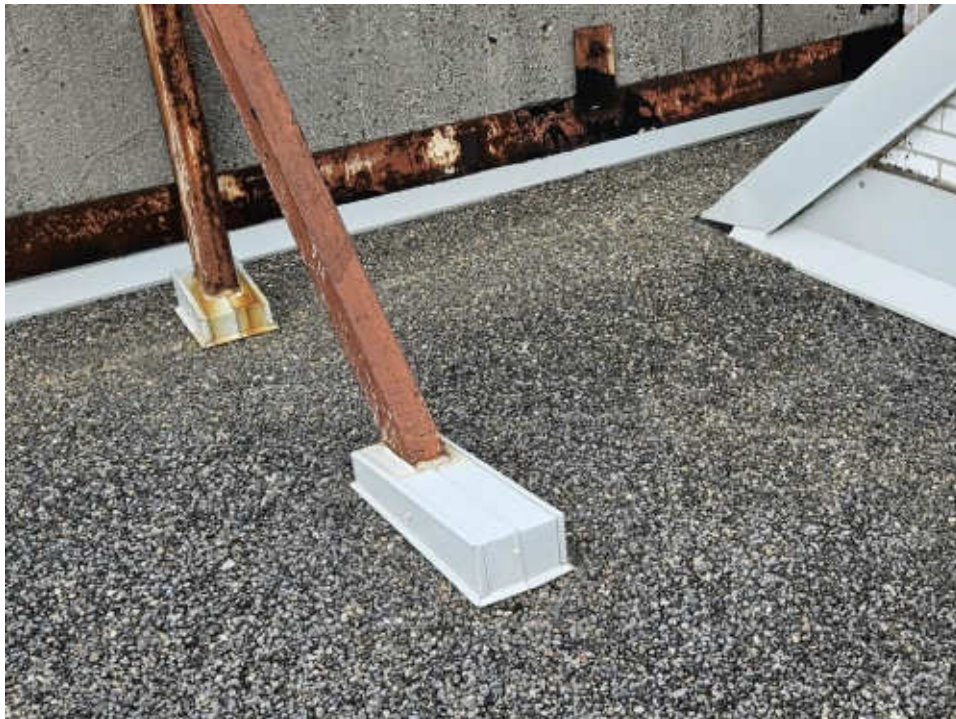
Photo #16: Example of Flashing over Precast Screen Structural Steel Support – BUR Section
