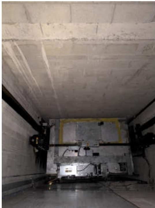
Photo #2: Passenger Elevator Car Top
