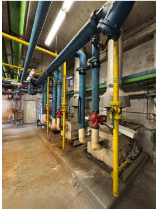
Photo #7: Gas Fired Heating Boilers
