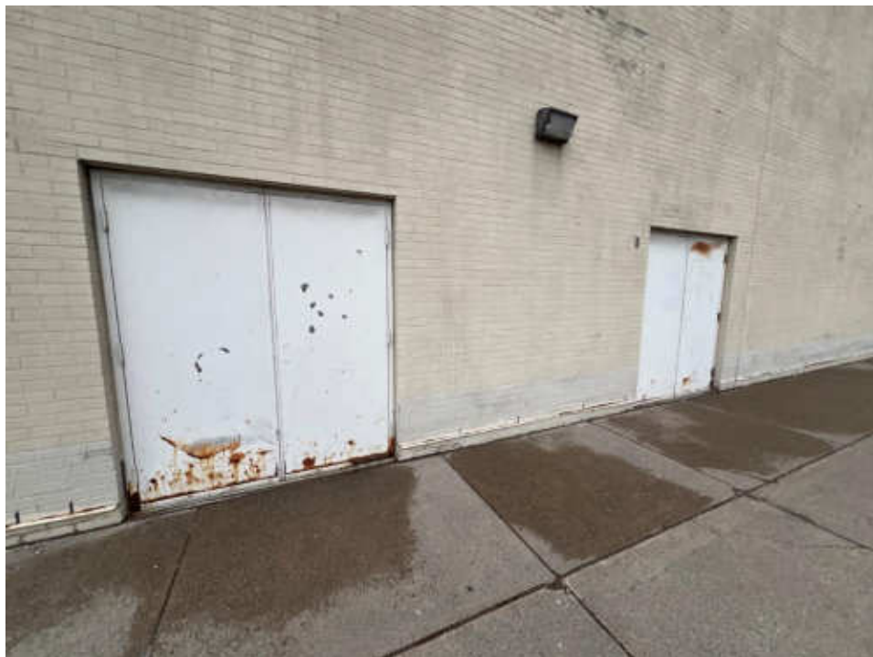
Photo #10: Typical Hollow Metal Service Doors
