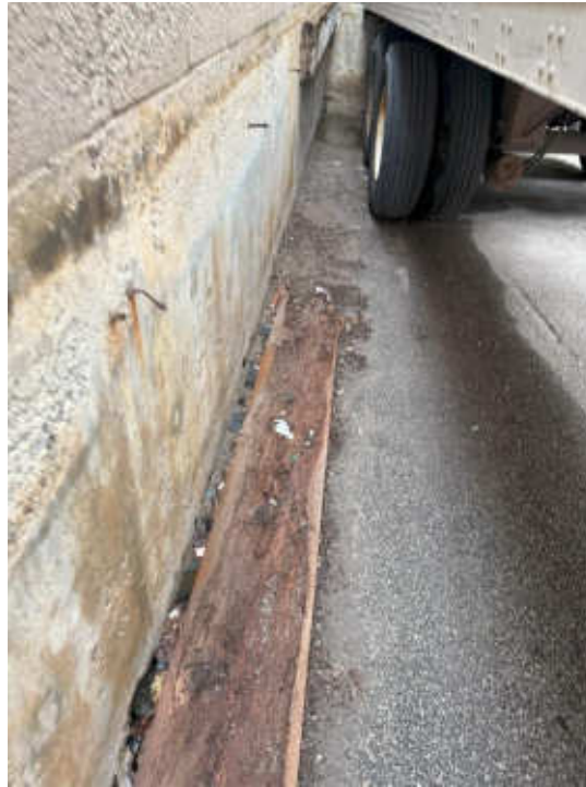
Photo #5: Loading Dock Area Retaining Wall. (Note deteriorated wood bumper guard on ground.)
