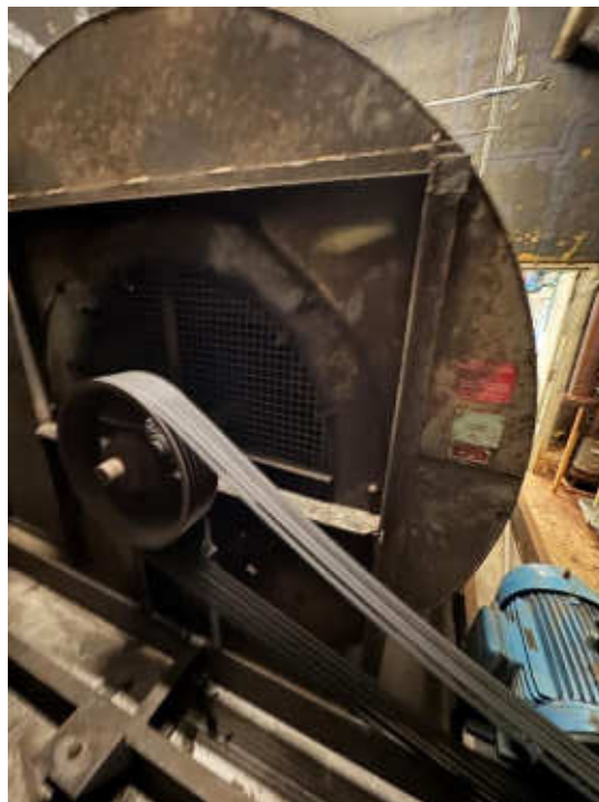
Photo #14: AHU-1 Supply Fan Belt Drive Motor
