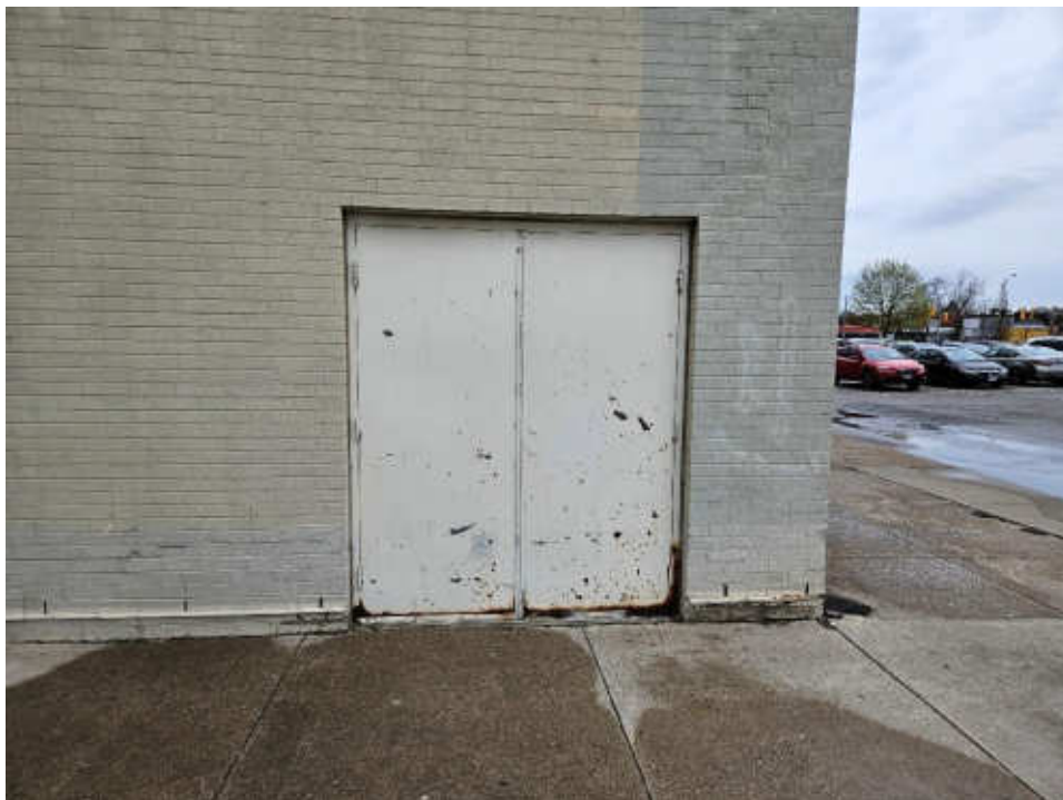
Photo #32: Example of Corrosion at Service Doors
