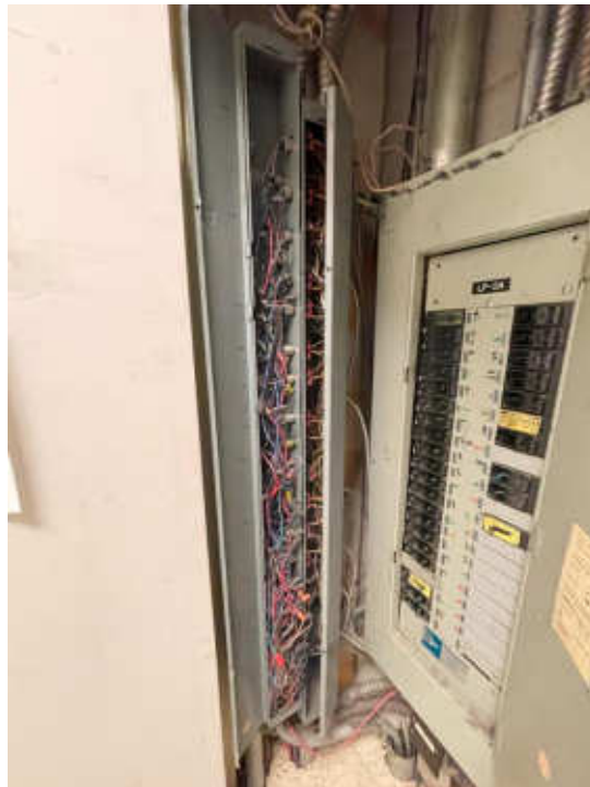
Photo #5: Lighting control relay panel
