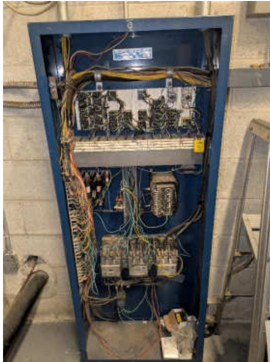
Photo #7: Freight Elevator Controller
