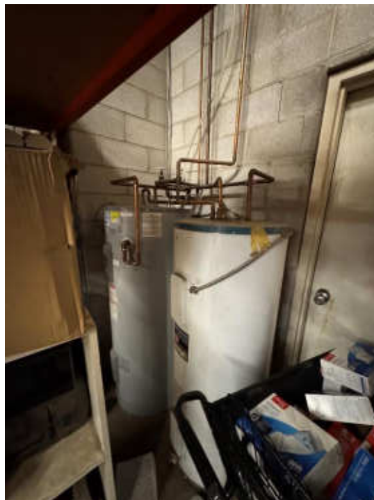
Photo #22: Electric Domestic Hot Water Heaters
