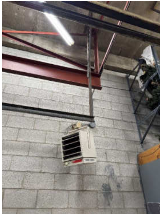
Photo #26: Loading Dock Electric Unit Heater
