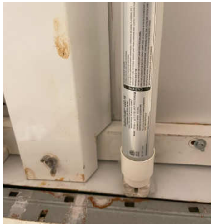
Photo #8: Retrofitted T8 bulbs inside old housing
