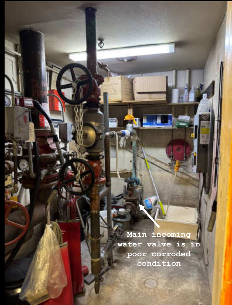
Fire Safety Systems - Main incoming water valve is in poor corroded condition
