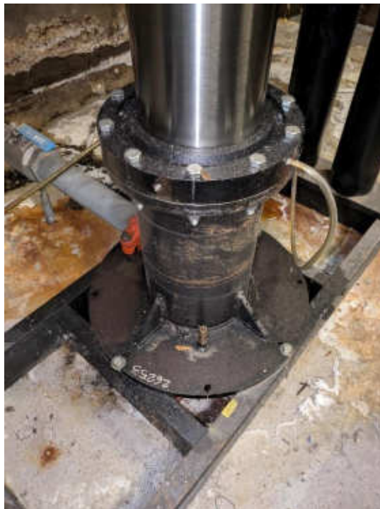
Photo #8: Freight Elevator Hydraulic Cylinder
