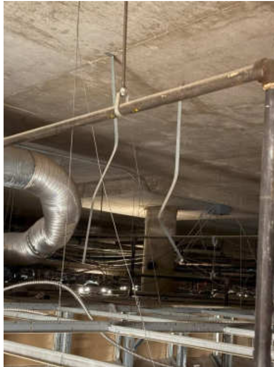
Photo #1: Underside Roof Slab Concrete Column and Drop Panel General Condition
