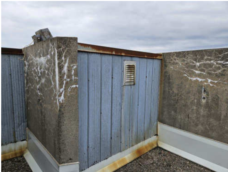
Photo #8: Metal Cladding at Roof Level
