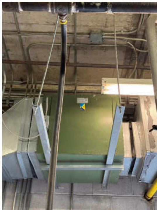
Photo #8: Combustion Air Intake Fan
