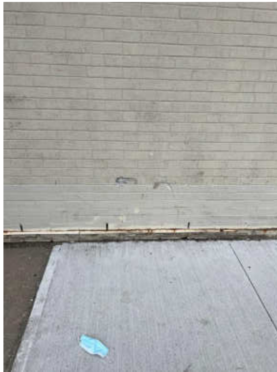
Photo #15: Damaged Brick at exterior cladding
