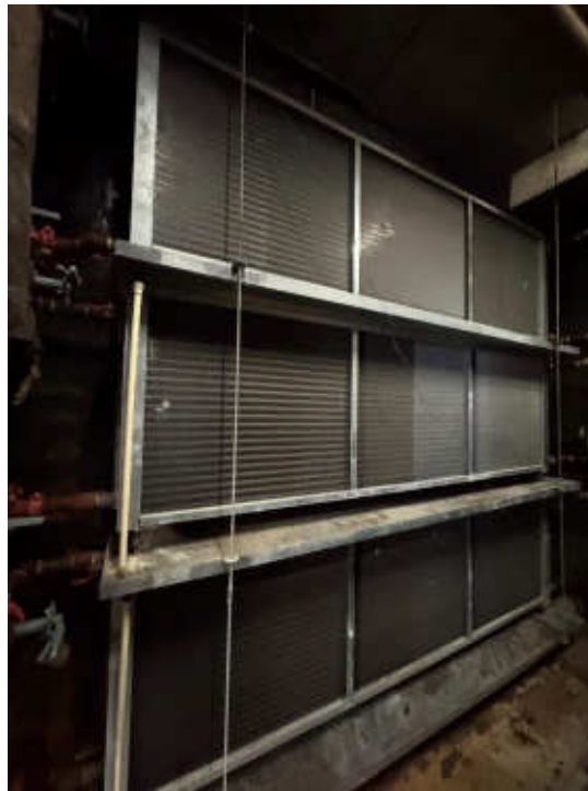
Photo #13: AHU-1 Dual Temperature Heating/Cooling Coil
