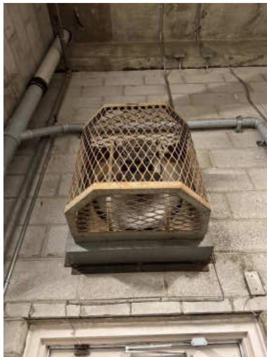
Photo #28: Garbage Room Wall-mounted Exhaust Fan
