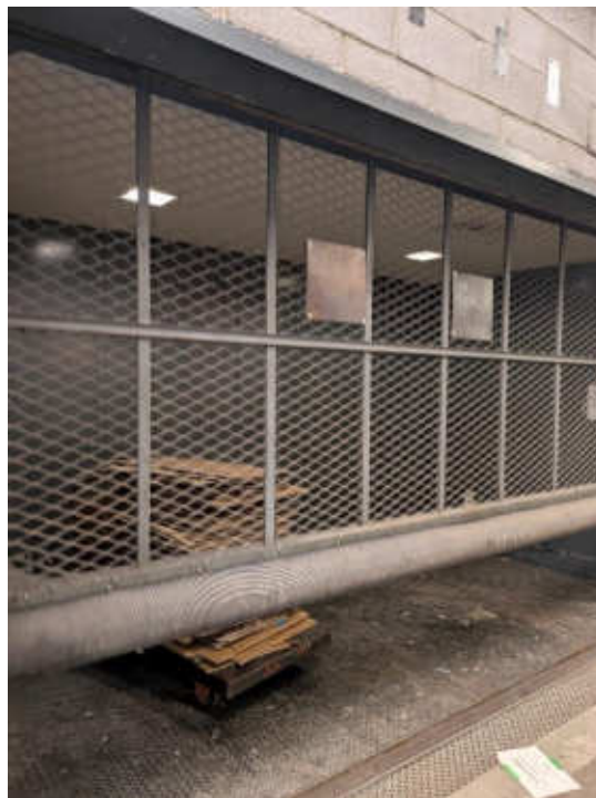
Photo #6: Freight Elevator Car Gate
