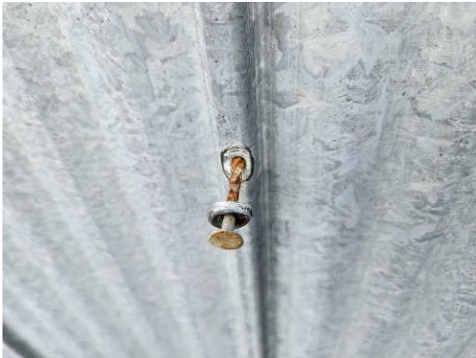
Photo #38: Backed Out and Corroded Fastener at Roof Level Metal Cladding
