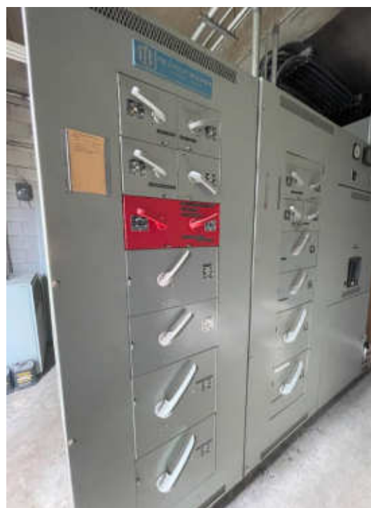
Photo #2: Main electrical switchboard
