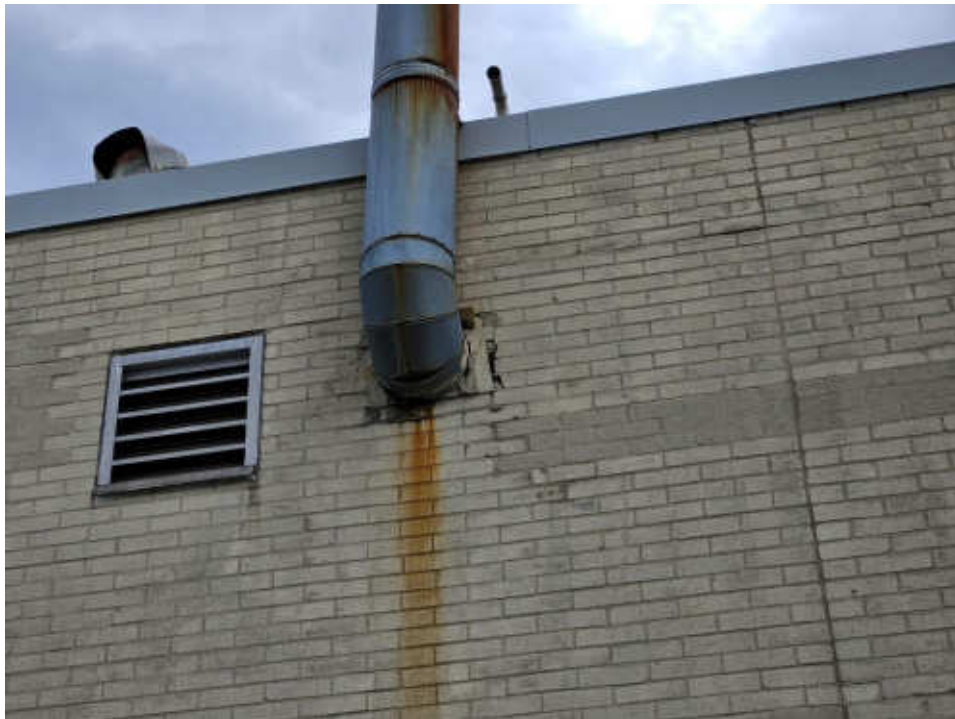
Photo #36: Damaged Brick and Unsealed Penetration
