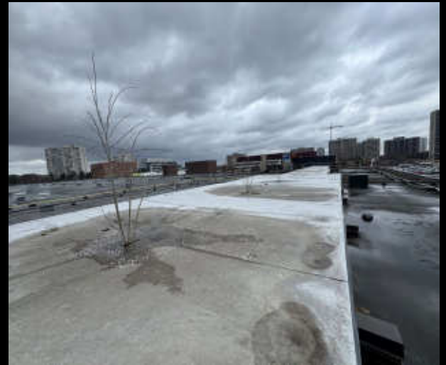
Condition of Roof - Lack to no maintenance causing ponding, poor drainage, vegetation growth
