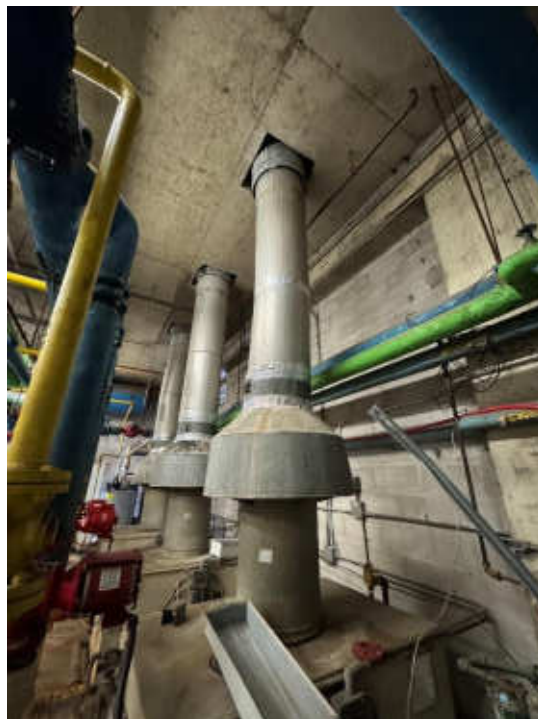
Photo #10: Heating Boilers Venting System
