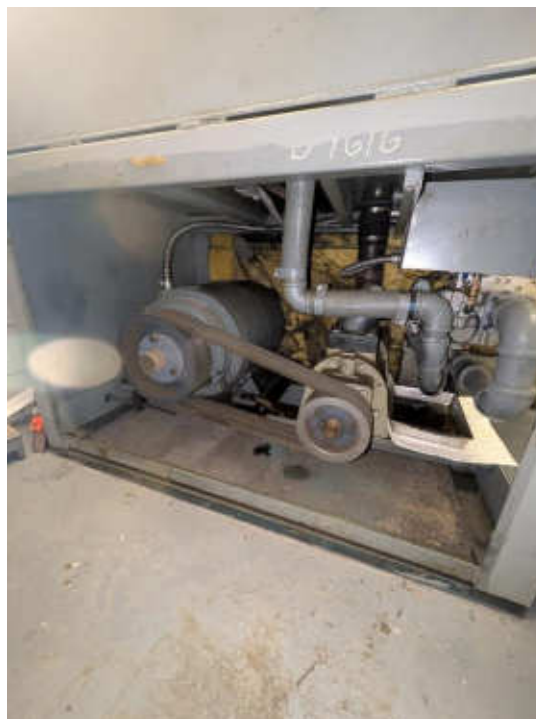
Photo #10: Freight Elevator Power Unit Pump
