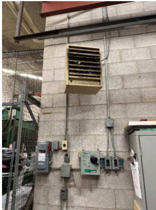
Photo #27: Loading Dock Electric Unit Heater
