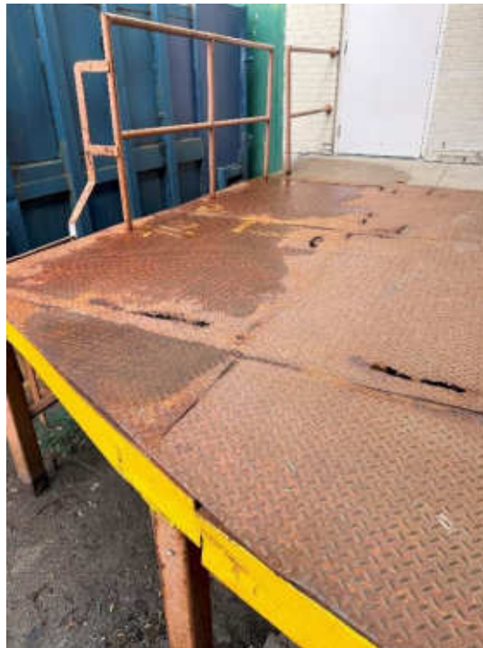
Photo #7: Top of Steel Loading Dock Extension (Note: Through corroded steel checker plate).
