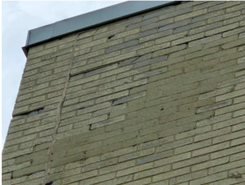
Photo #13: Example of Spalled, Cracked and Deteriorated Brick/Mortar Joints at Roof Level
