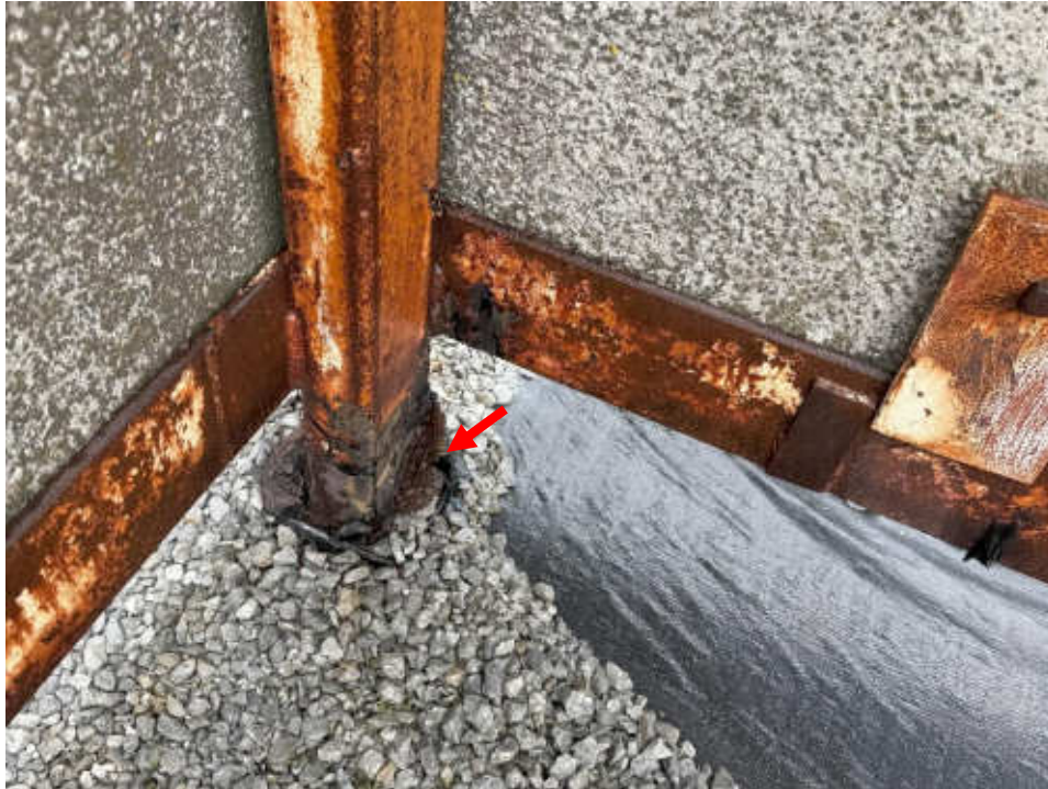
Photo #28: Typical Corrosion at Structural Framing for Roof Level Precast Screen. Potential Section Loss at Roof Pitch Pocket Flashing Detail
