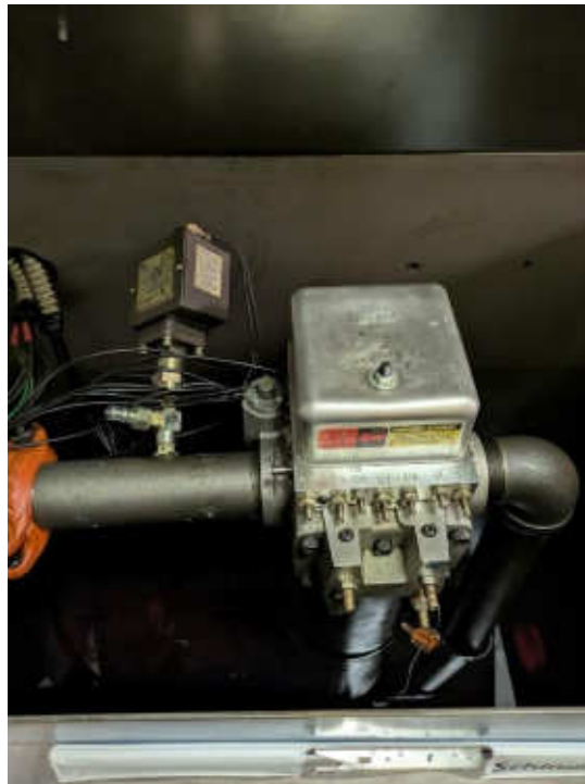
Photo #3: Passenger Elevator Control Valve
