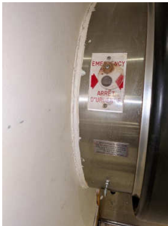
Photo #12: Escalators Emergency Controls
