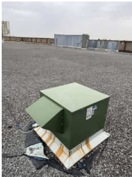
Photo #20: Rooftop Washroom Exhaust Fan
