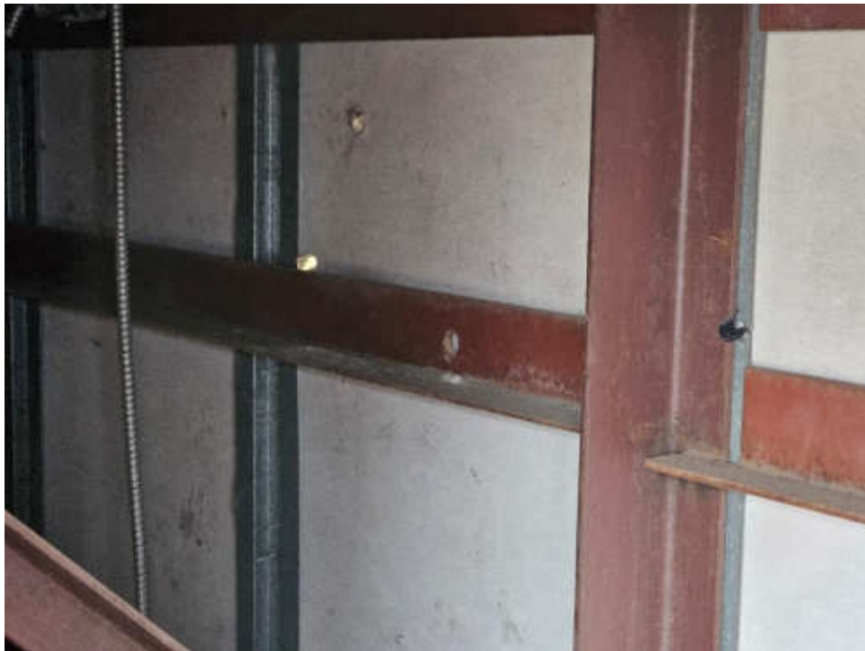
Photo #34: Daylight Visible from Unsealed Penetration at Interior Space
