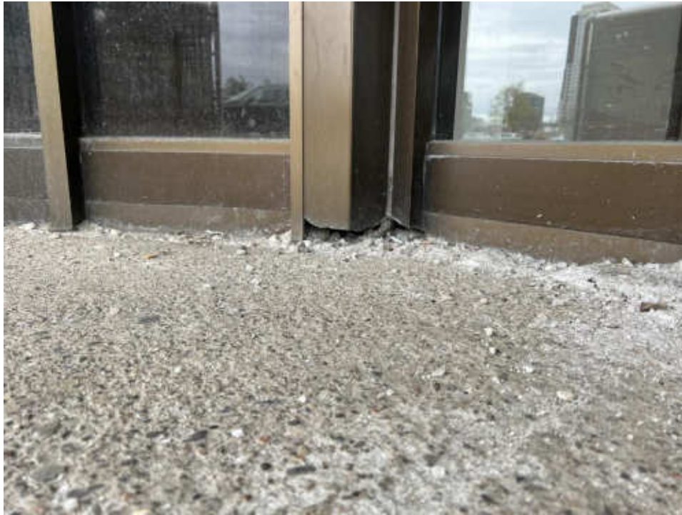
Photo #31: Corrosion at Base of Main Entrance Framing
