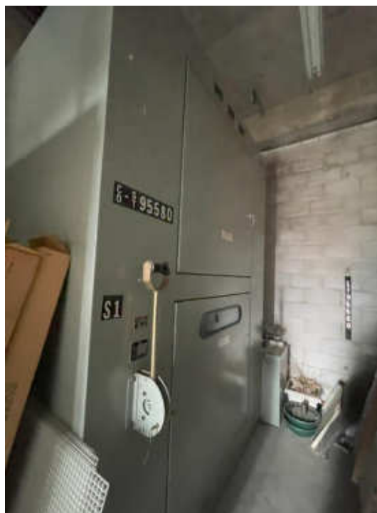
Photo #1: Main HV switch
