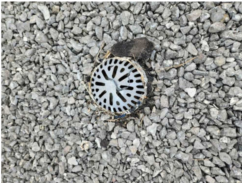
Photo #8: Typical Roof Area Drain
