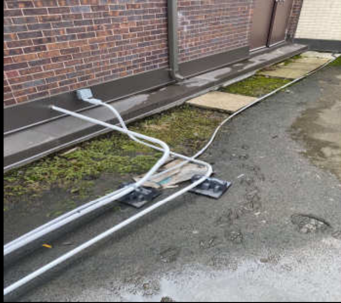
Condition of Roof - Lack to no maintenance causing ponding, poor drainage, vegetation growth
