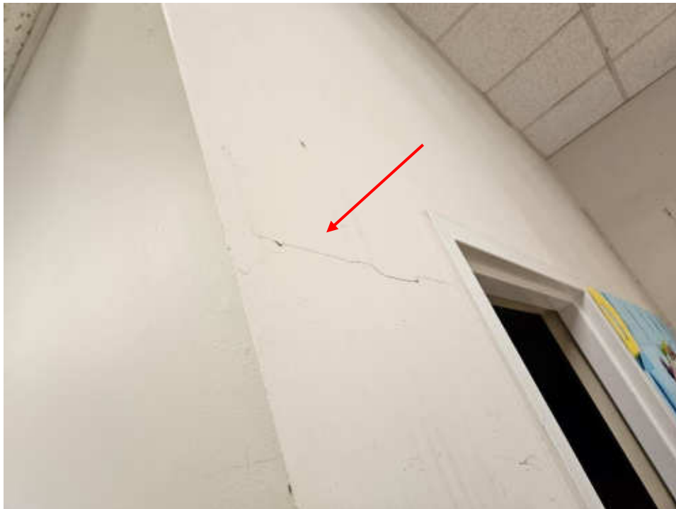
Photo #16: Cracked Finishes in Second Floor Office Area
