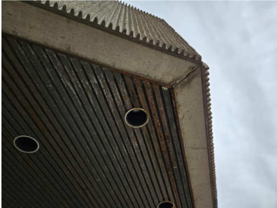
Photo #18: Corrosion and Moisture Deterioration at Main Entrance Soffit
