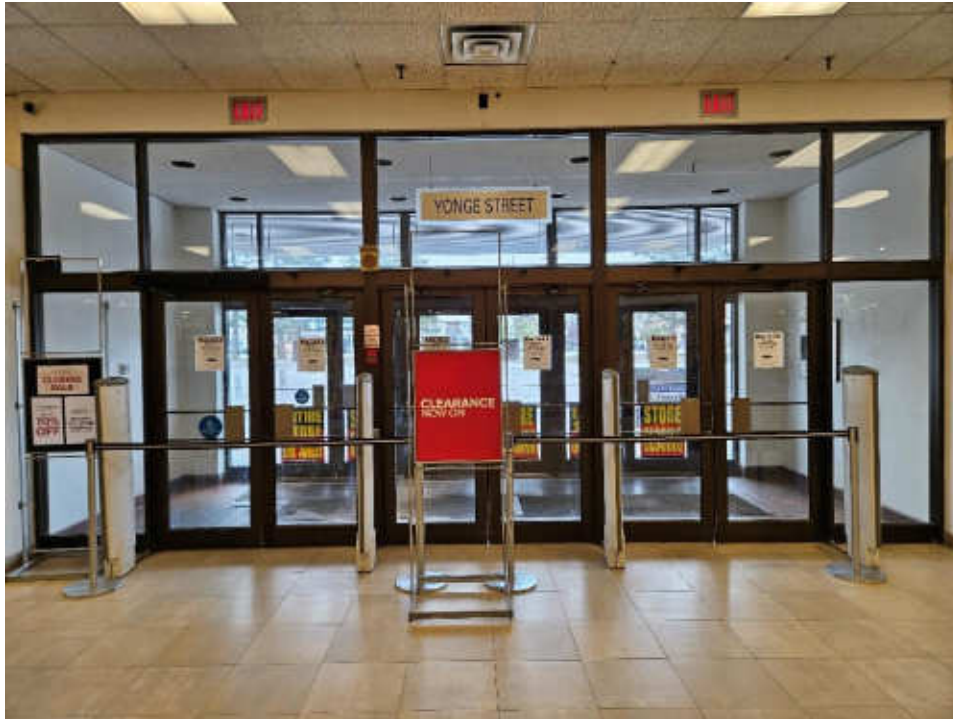
Photo #5: Typical Single Glazed Vestibule Interior Partition
