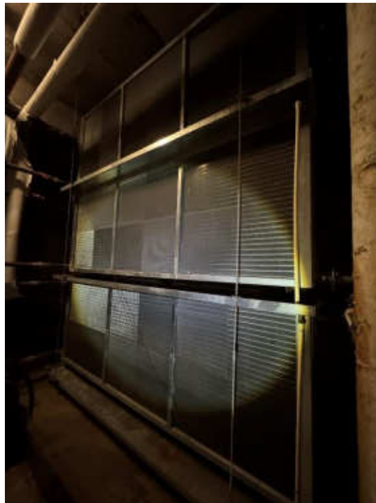
Photo #18: AHU-2 Dual Temperature Heating/Cooling Coil
