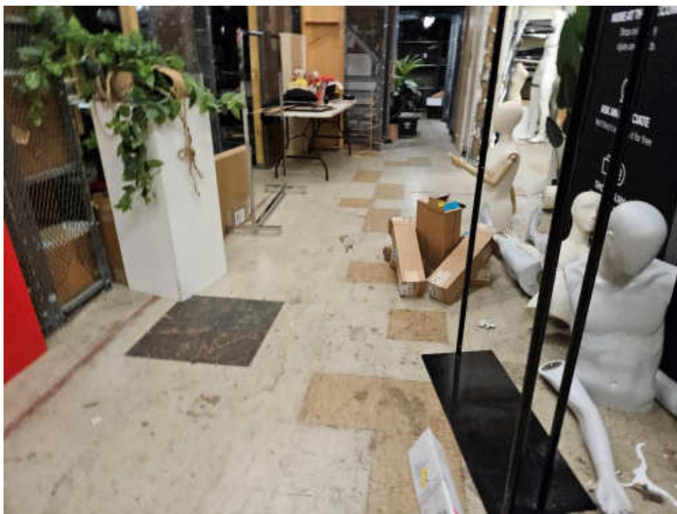
Photo #13: Example of Vinyl Tile Condition
