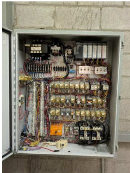
Photo #4: Passenger Elevator Controller
