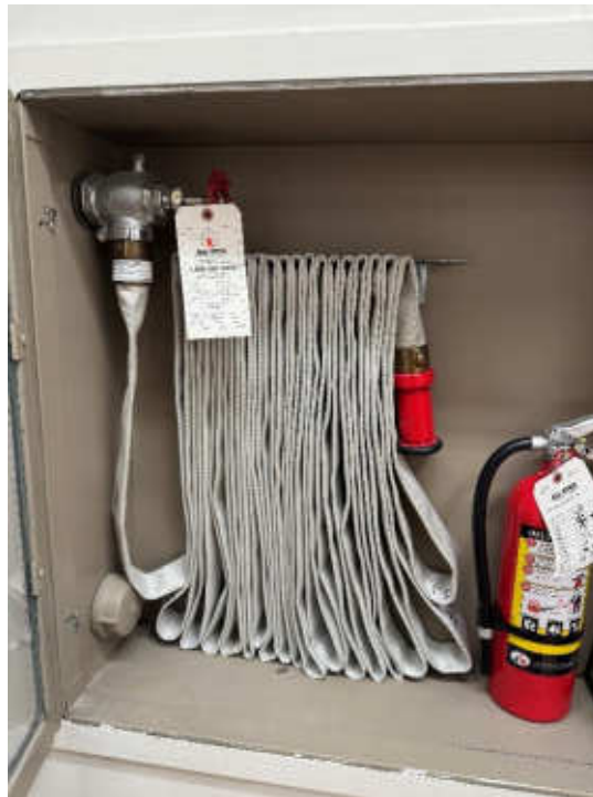
Photo #35: Typical Fire Hose Cabinet
