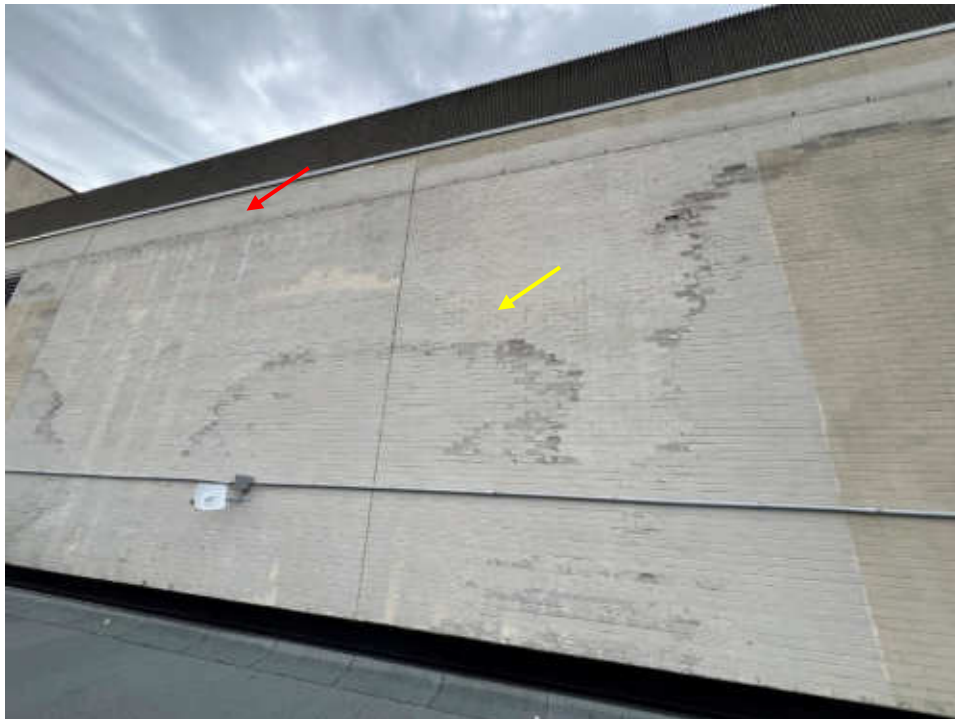
Photo #20: Overview West Elevation, Deteriorated Brick Coating (Yellow) and Efflorescence (Red)
