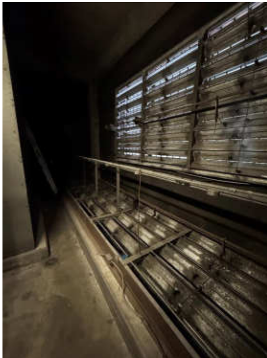
Photo #16: AHU-2 Mixing Air Plenum
