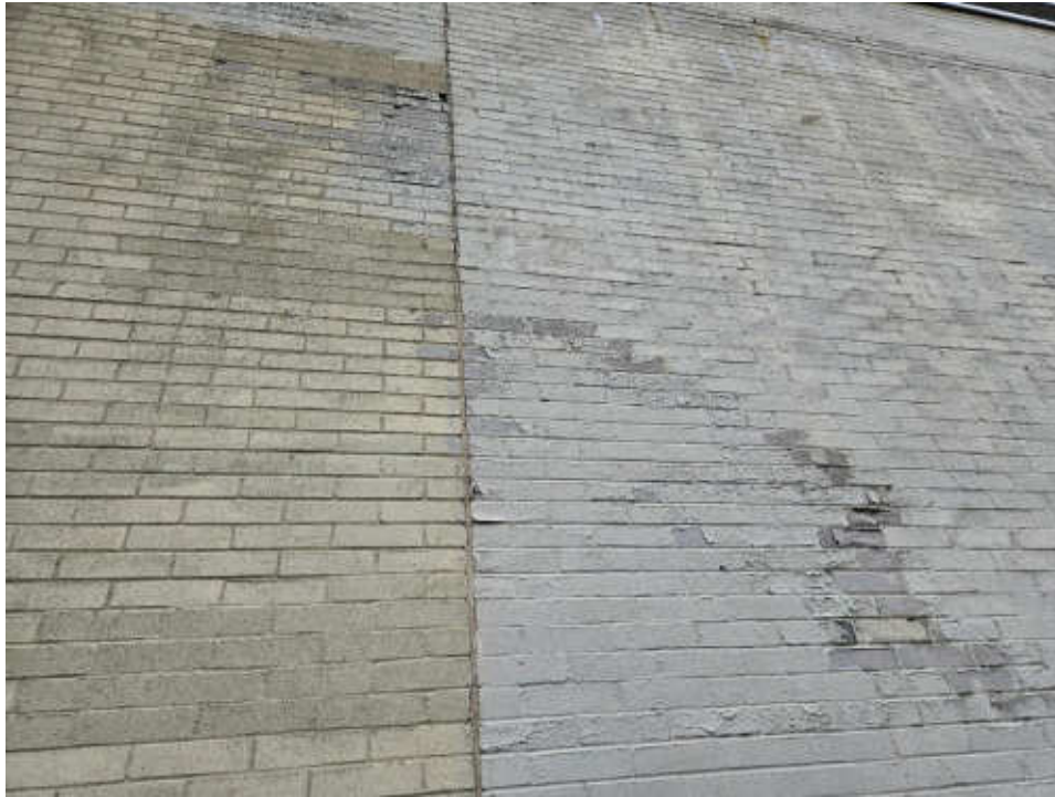
Photo #19: Overview of Different Vintage and Colour Coatings and Peeling
