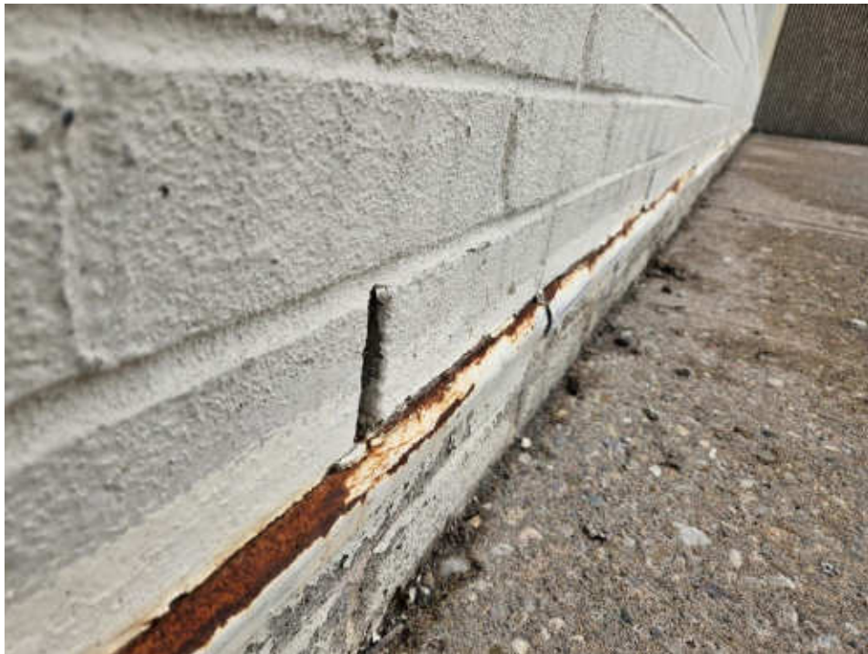
Photo #22: Typical Corroded Metal Drip Edge Flashing
