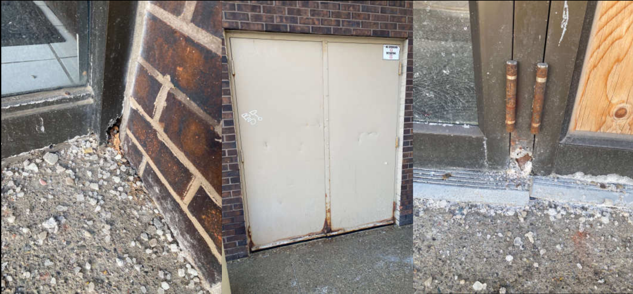
Exterior - Corrosions/Damages to Entrance and Egress doors
