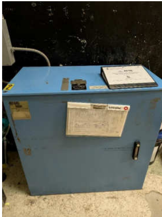
Photo #5: Passenger Elevator Power Unit and Tank
