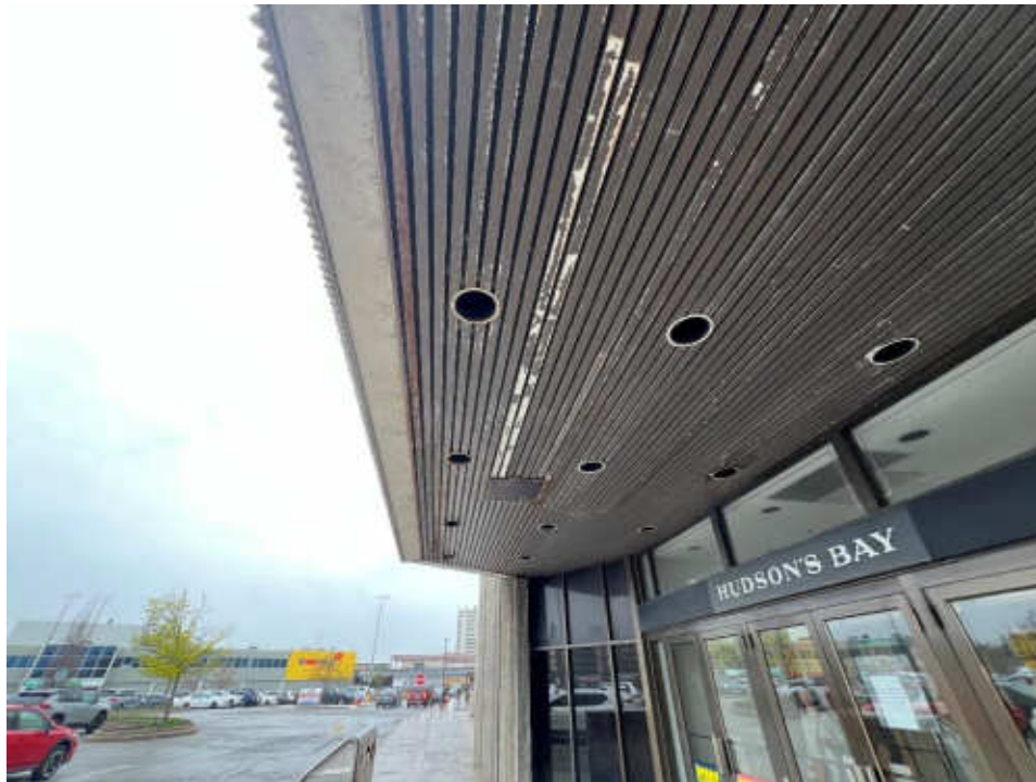
Photo #7: Typical Metal Soffit at Entrance
