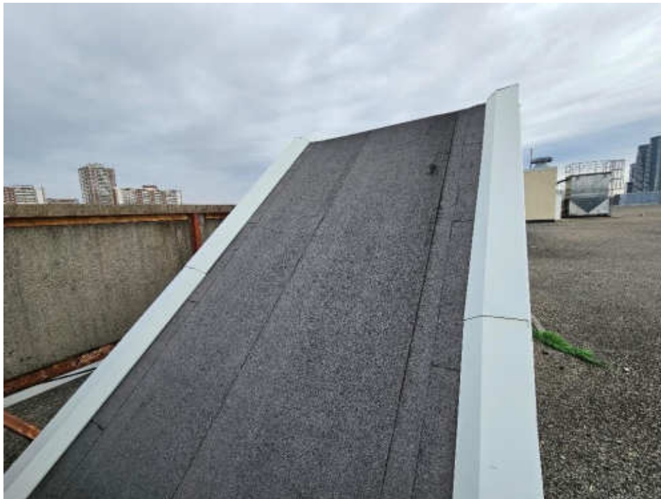
Photo #5: Overview of MBM membrane over Roof Stairwell
