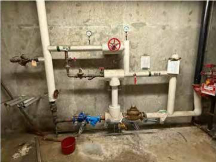
Figure 22. Domestic Water Assembly
