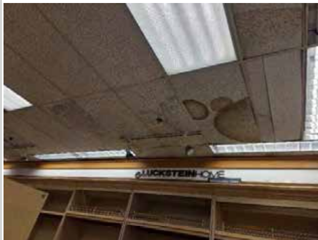
Photo 4 - Water stains on ceiling tiles
