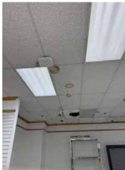
Figure 21. Water Leakage West Side (2 nd floor)
