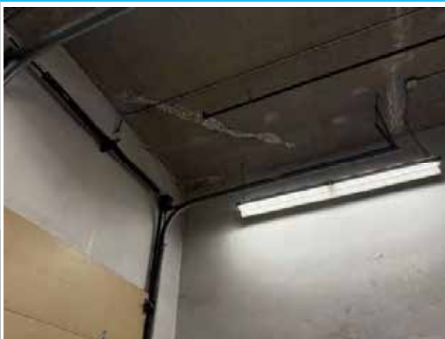
Photo 5 - Efflorescence on loading bay soffit
