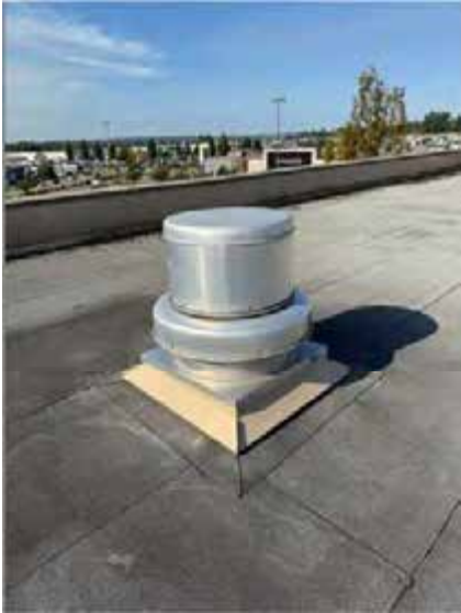
Figure 9. Washroom Exhaust Fan (EF-1)
