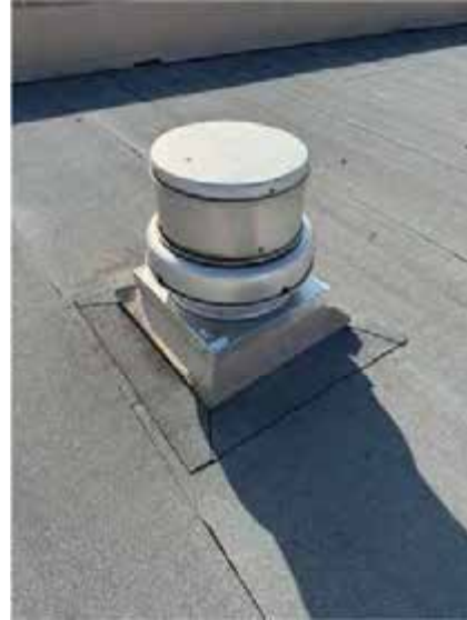
Figure 10. Electrical Room Exhaust Fan (EF-12)
