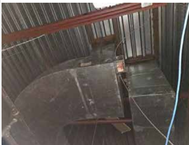
Photo 3 - Bare steel angles at mechanical penetrations through the steel deck
