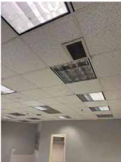
Figure 15. Typical Exhaust Grille Plugged by Dust
