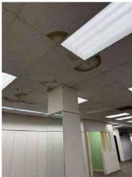
Figure 20. Water Leakage East Side (2 nd floor)
