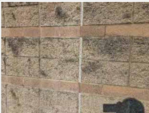
Photo 16 - Sealant joint in brick veneer
