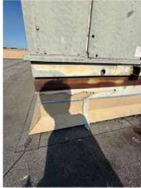
Figure 6. Roof Curb (Seal Damaged)
