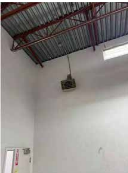
Figure 18. Typical Unit Heater
