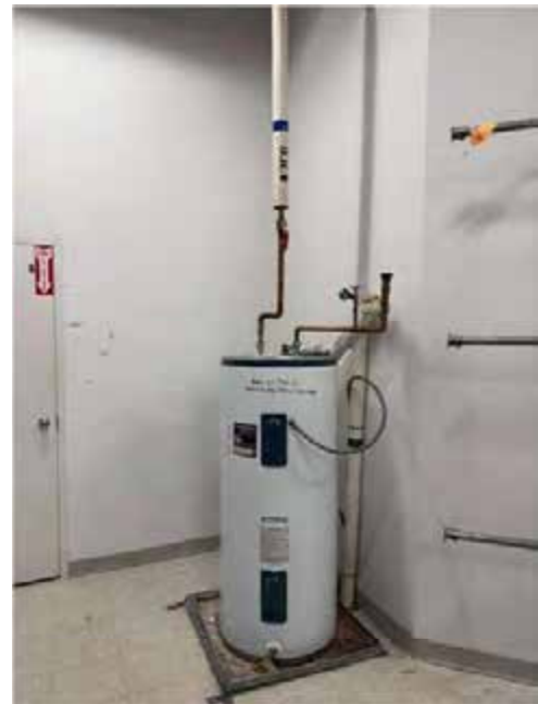
Figure 25. Typical Floor Mounted DHWT
