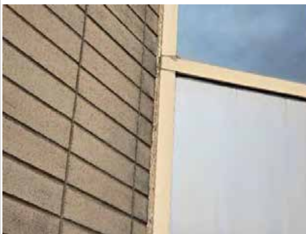
Photo 17 - Sealant joint between brick and curtain wall
