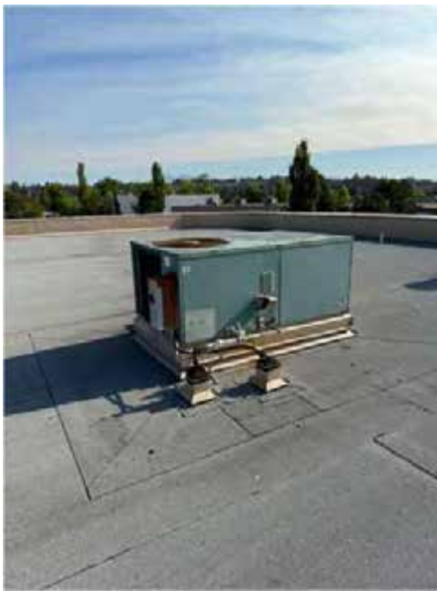
Figure 7. Roof Top Unit (AC-5)
