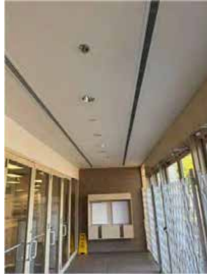
Figure 14. Typical Linear Diffuser
