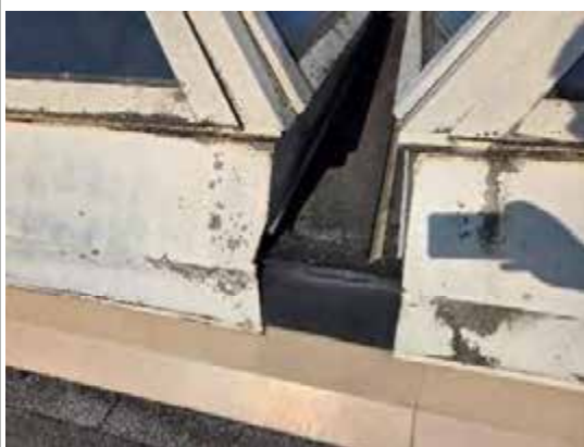
Photo 3 - 'Gutter' between skylights
