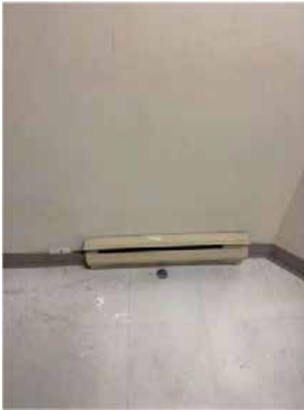
Figure 16. Typical Electric Baseboard Heater
