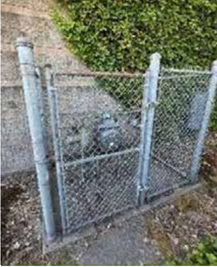
Figure 33. Natural Gas PRV & Meter
