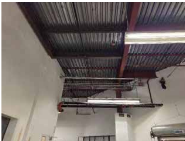
Photo 2 - Steel deck, open web steel joists, structural steel beams and columns
