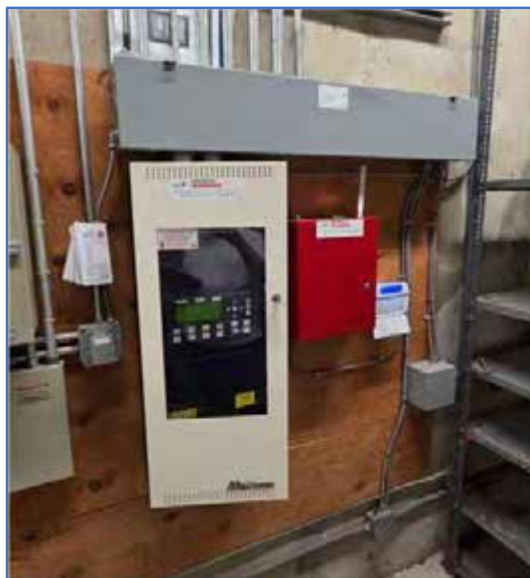
Picture 2 Mircom FX-2000 Fire Alarm Control Panel
