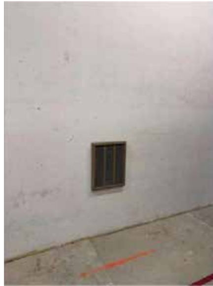
Figure 17. Typical Wall Cabinet Heater
