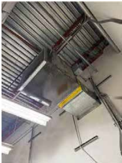
Figure 11. Elevator Machine Room Exhaust
