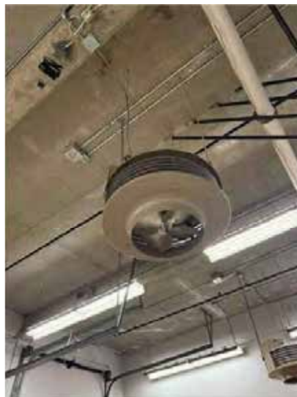
Figure 19. Typical Fan Coil Heater
