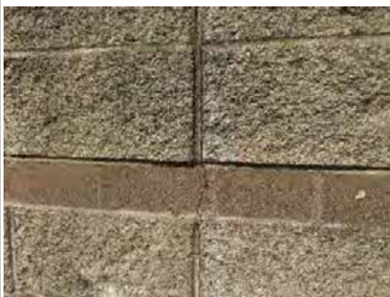
Photo 12 - Cracks in mortar between bricks
