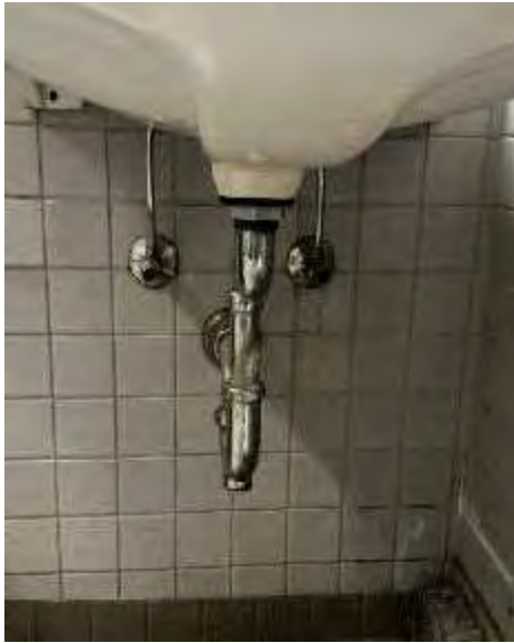
Figure 29. Sanitary Pipe Below Lavatory
