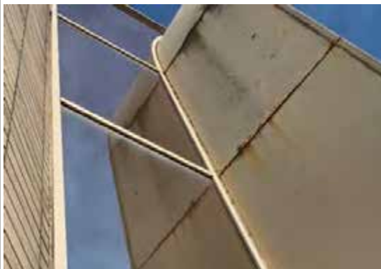
Photo 15 - Corrosion of metal panels
