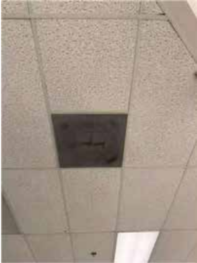
Figure 13. Typical Perforated Supply Diffuser
