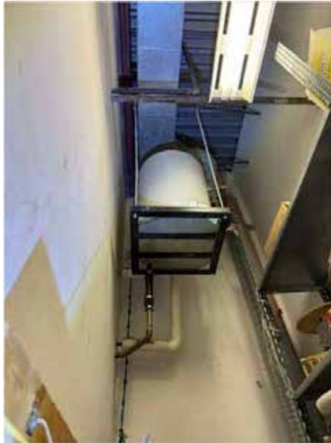
Figure 26. Typical Ceiling Mounted DHWT
