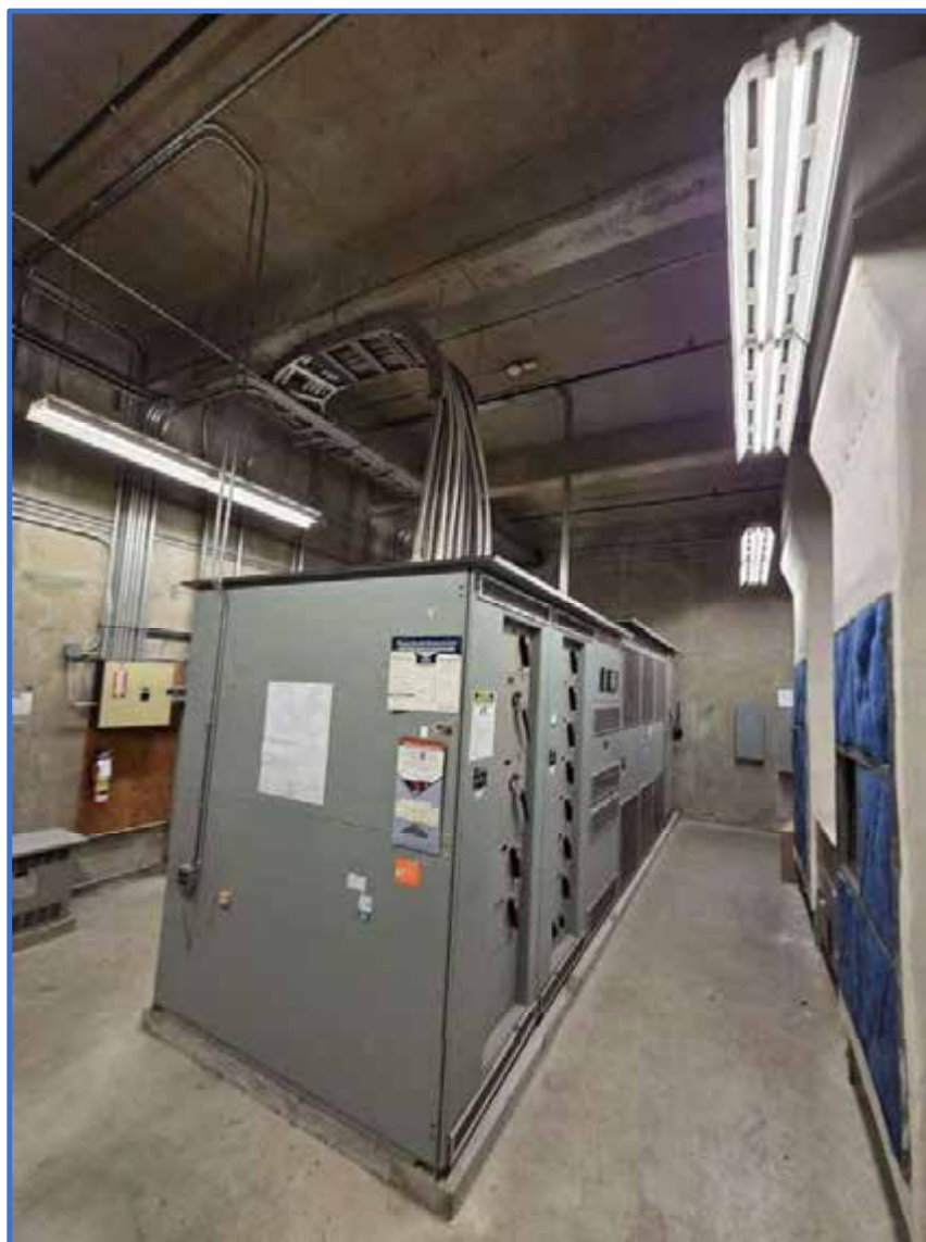
Picture 1 Main Distribution Center with Electrical Room #1 (w/ 1000kVA transformer, metering cubicle and secondary distribution)
