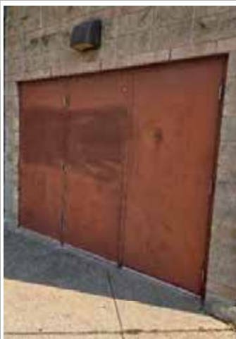
Photo 20 - Typical hollow metal service door
