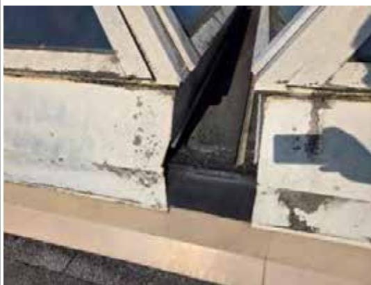
Photo 9 - Gutter between skylights
