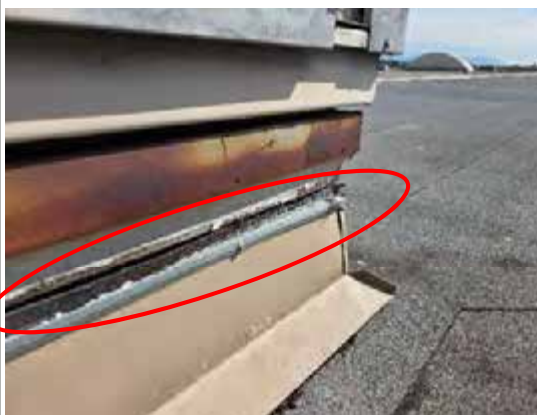
Photo 2 - Damaged transition membrane at roof curb
