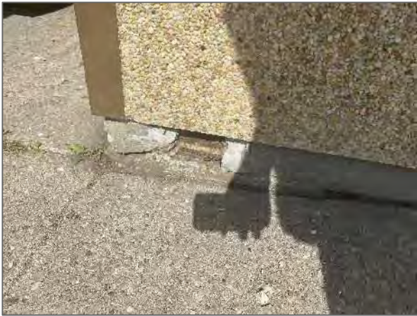
View of delaminated concrete in the cast-in-place concrete foundation wall noted on the east elevation of the Site Building.
