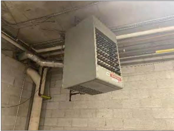
View of a typical suspended unit heater.
