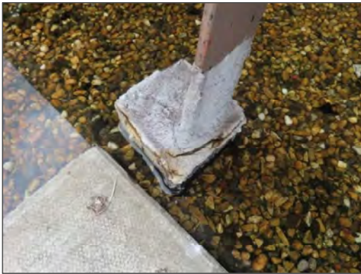
View of deteriorated pitch pocket serving the ladder footing atop Section 8 of the Site Building.
