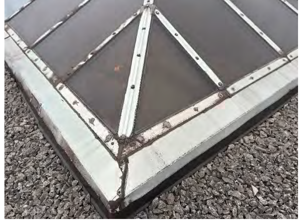
Figure 10: Deteriorated face sealant observed at skylight.
