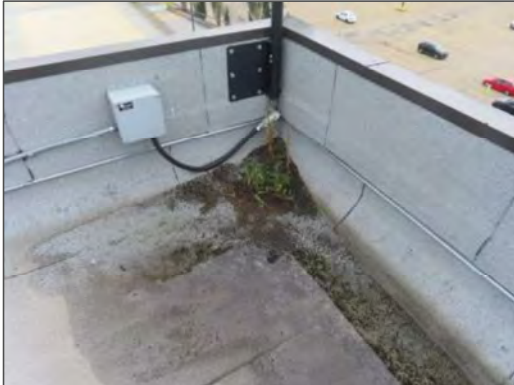
View of typical degranulation and deterioration of the modified bitumen membrane atop multiple Sections of the Site Building.
