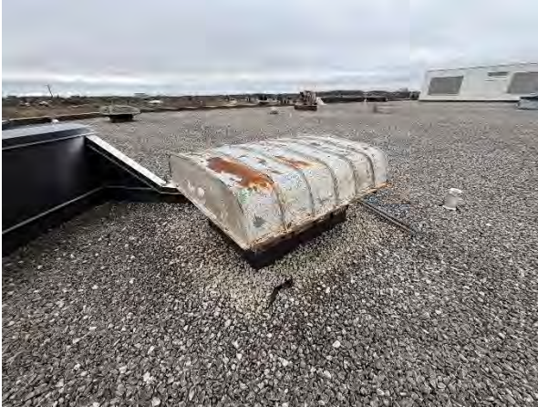
Figure 5: Exhaust hoods are typically corroded.
