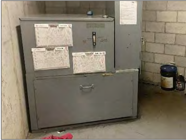
View of the hydraulic reservoir.
