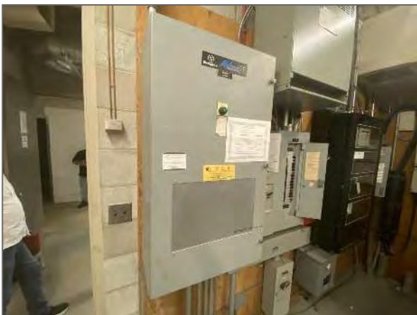
View of the "Westinghouse" automatic transfer switch.
