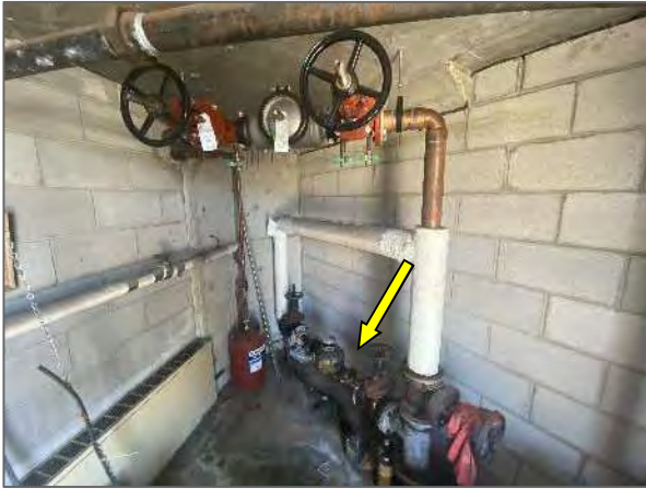
View of the domestic water main incoming line.
