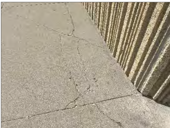
View of typical cracking in the cast-in-place concrete walkways noted to the east of the Site Building.
