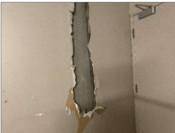
View of typical damaged gypsum wall board noted in the stairwell in the southeast portion.
