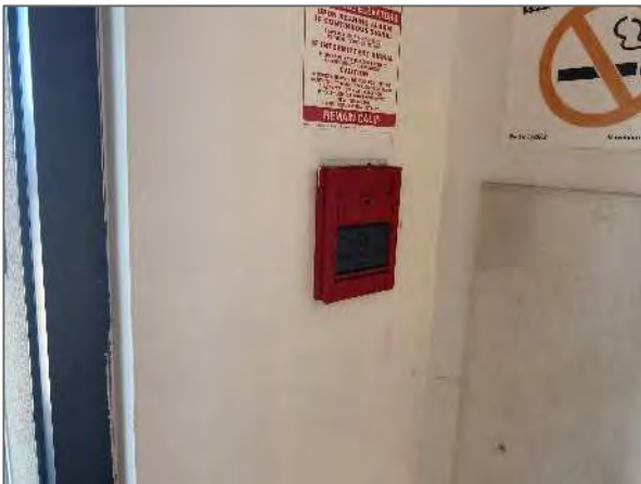
View of a typical manual pull station.
