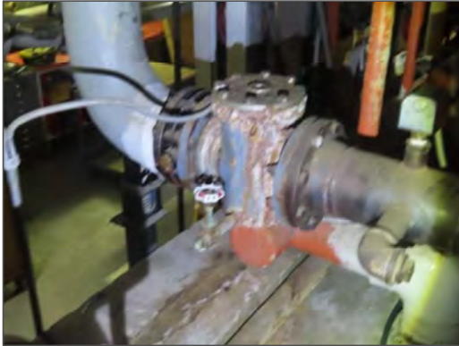
View of typical corrosion and calcium build up on piping fittings within the 2 nd floor mechanical room of the Site Building.
