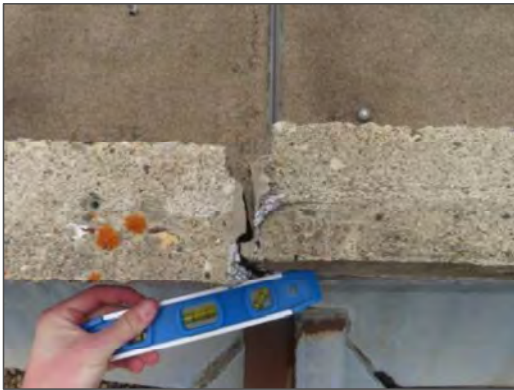
View of typical minor movement noted on precast concrete panels on multiple elevations the Site Building.
