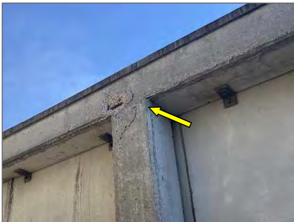
View of a typical bent/impact damaged steel column noted within the warehouse area of the Site Building.
