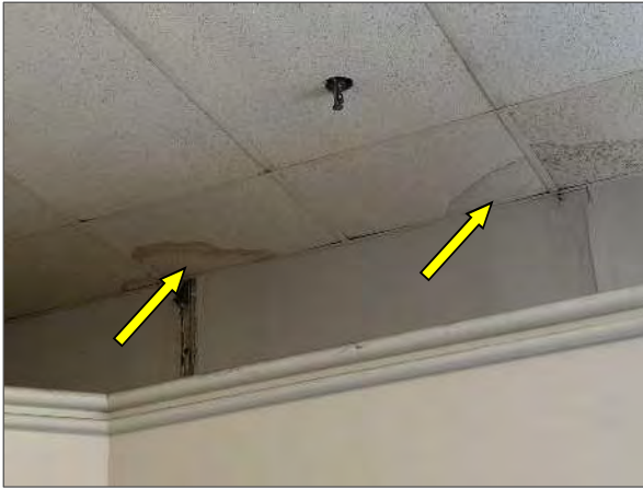
View of moisture/water-stained ceiling tiles noted adjacent to the south entrance of the Site Building.
