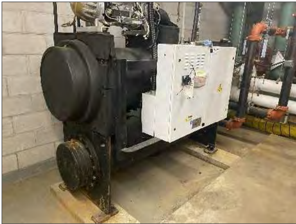
View of a "Smardt" chiller.
