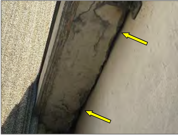
View of deteriorated concrete noted on a reinforced concrete beam in the southeast portion above the secondary roof.
