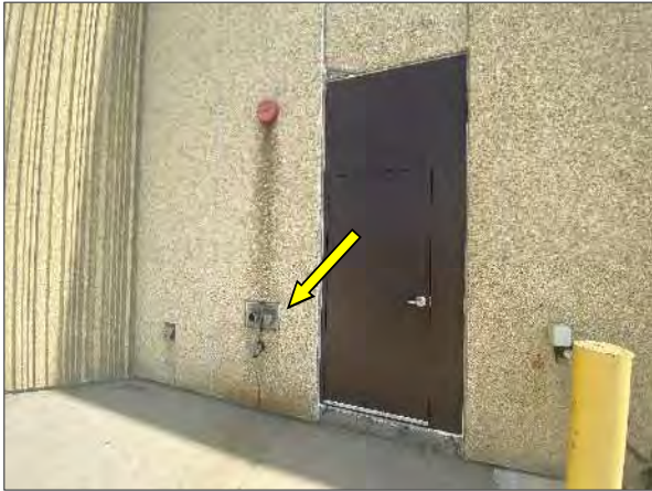
View of the fire department connections located on the south elevation of the Site Building.
