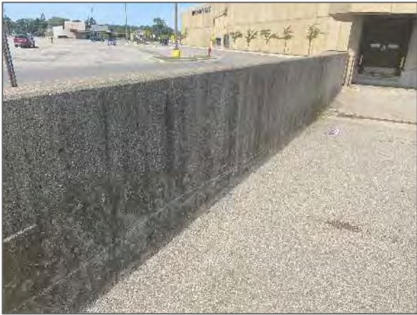
View of a typical cast-in-place retaining wall serving the shipping/receiving area.
