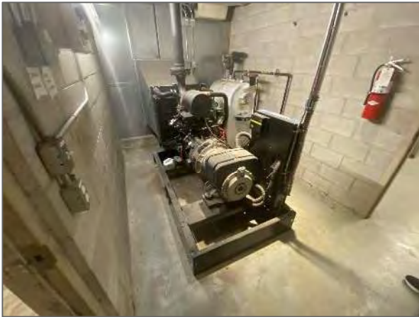
View of the "SDMO" diesel-fired emergency generator.
