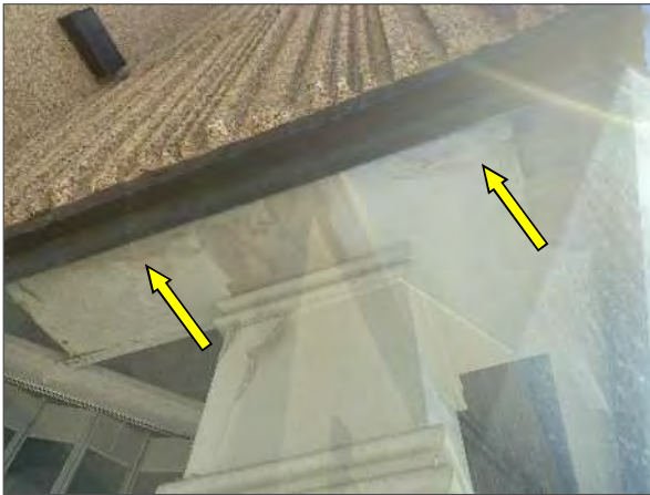
View of water damage in the gypsum wall and ceilings boards, reportedly due to a previous pipe leak noted adjacent to the south entrance of the Site Building.
