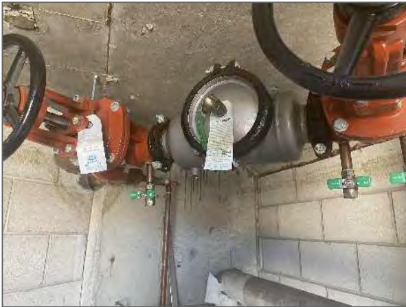
View of the "Zurn Wilkins" backflow prevention device installed onto the domestic water main incoming line.
