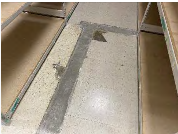
View of damaged/missing vinyl floor tiles noted on the second floor of the Site Building.
