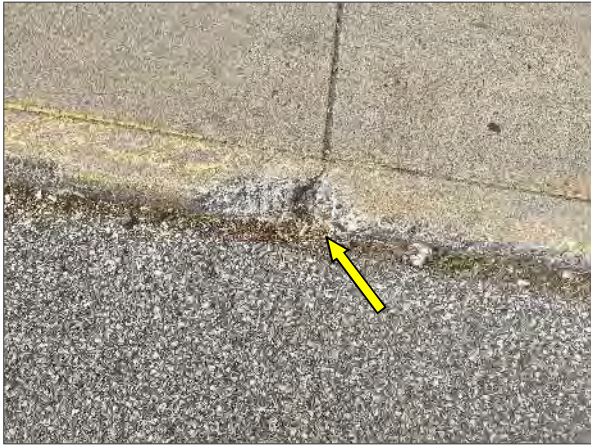
View of typical deterioration in the concrete curbs noted to the east of the Site Building.
