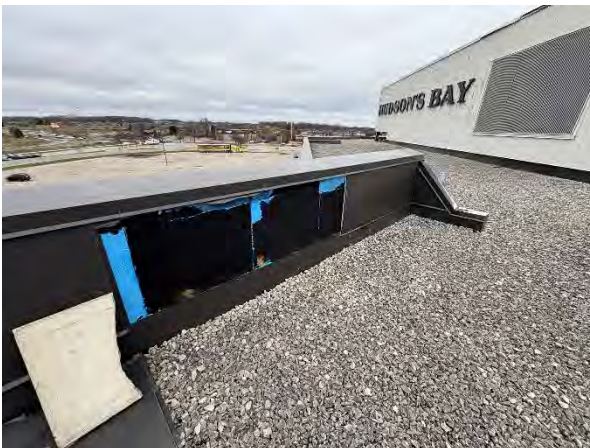
Figure 7: Missing parapet cladding removed, exposed membrane flashing.
