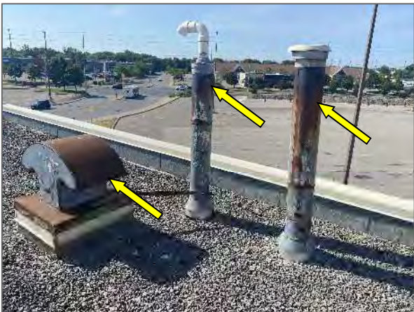
View of corrosion noted on the combustion and exhaust vents on the south portion of the Site Building.
