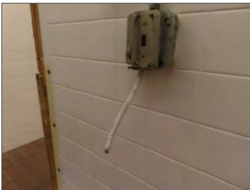
View of exposed wires within the kitchen area on the 2 nd floor of the Site Building.
