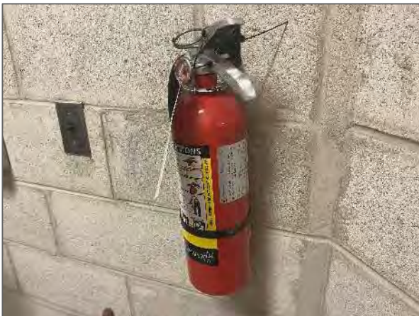
View of a typical standalone "dry" chemical fire extinguisher.
