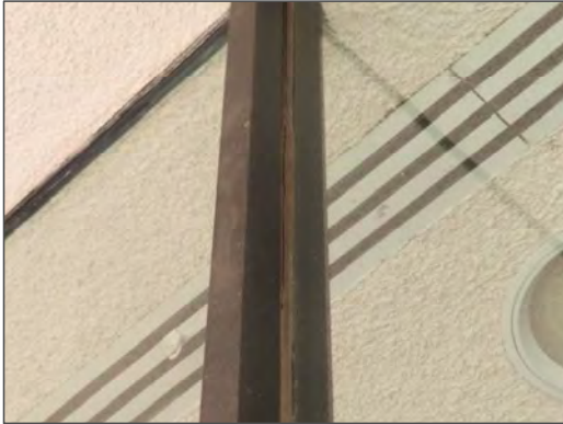
View of window sealant deterioration on the east elevation the Site Building.
