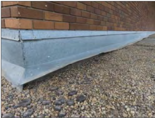
View of typical area of lifted flashing on the north portion atop Section 8 of the Site Building.
