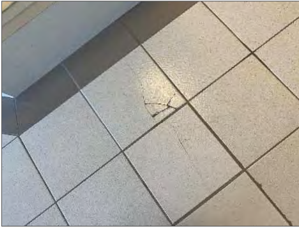
View of typical cracked/broken ceramic floor tiles noted in the west portion of the first floor of the Site Building.
