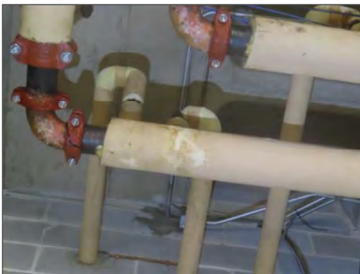
View of typical moisture stained piping insulation observed within various mechanical rooms of the Site Building.
