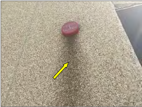
View of typical moisture staining noted on the south elevation of the Site Building.
