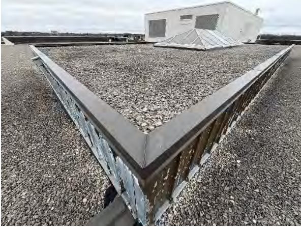
Figure 9: Peeling paint finish at metal siding.
