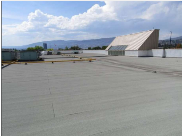
General view of a typical modified bitumen membrane Roof Section A2 serving the Site Building.
