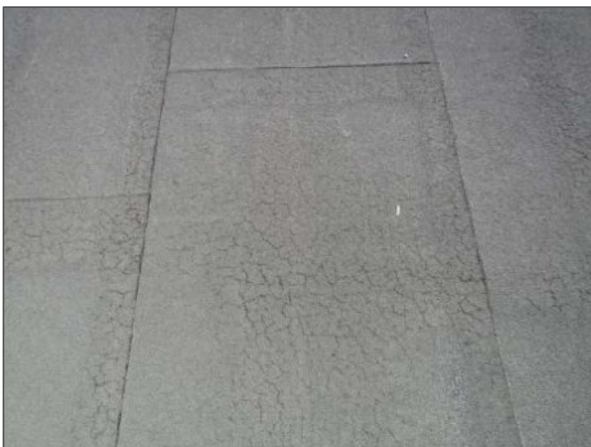
Areas of membrane crazing of the modified bitumen membrane roof system were noted atop Roof Section A3 in multiple locations.
