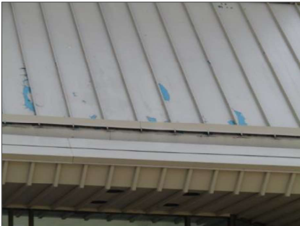
Areas of delaminated paint were noted atop the sloped metal mansard style roof areas.
