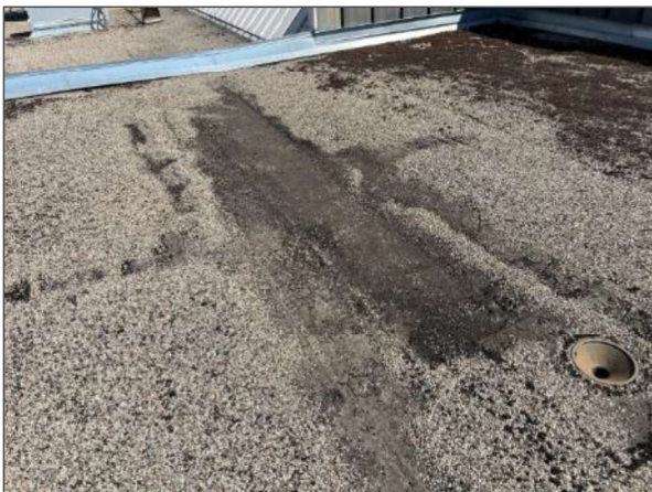
Areas of exposed membrane and previous repair work to the BUR system serving Roof Section 6 were observed.
