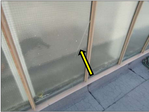
Cracked glazed units serving the glazed roof noted on the west portion of the Site Building were observed.
