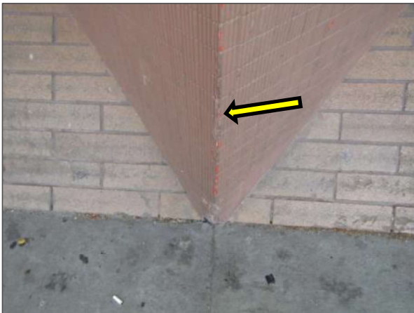
Damaged clay wall tile was noted on the west elevation.
