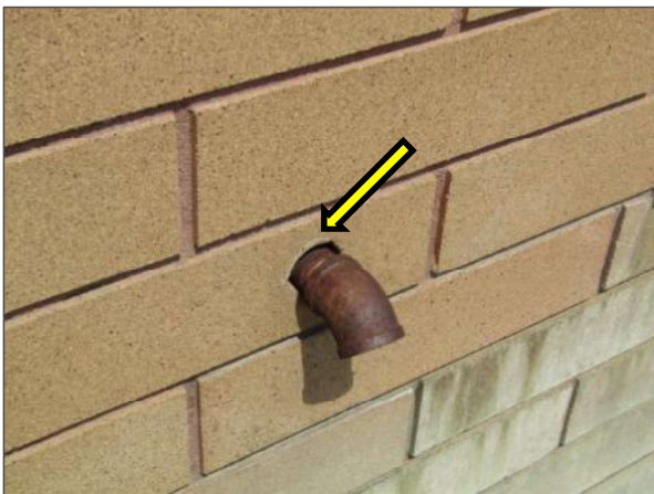
An unsealed wall penetration was noted on the south elevation.
