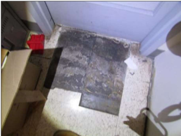
Damaged vinyl flooring was noted in multiple locations of the Site Building.
