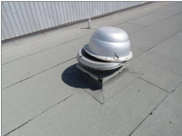
Damaged exhaust units were noted atop the Site Building.
