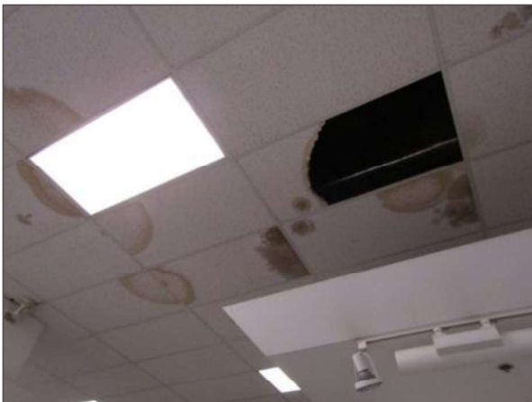
Missing/damaged/moisture stained ceiling tiles were noted in multiple locations of the Site Building.
