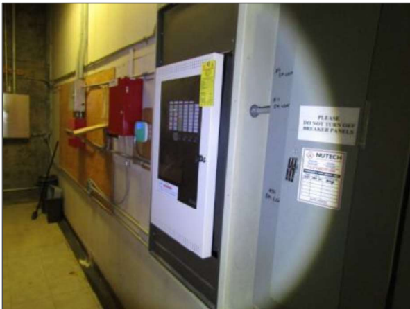
General view of the "Mircom" main fire alarm panel.
