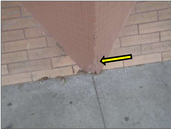
Damaged clay wall tile was noted on the north elevation.
