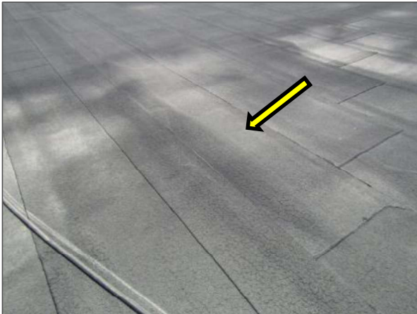
Areas of membrane blistering of the modified bitumen membrane roof system were noted atop Roof Section A4 in multiple locations.
