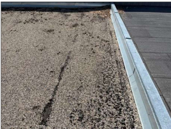
Areas of asphalt bleed through were noted atop the BUR system serving Roof Section 6.
