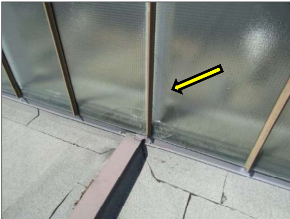
Cracked glazed units serving the glazed roof noted on the north portion of the Site Building were observed.
