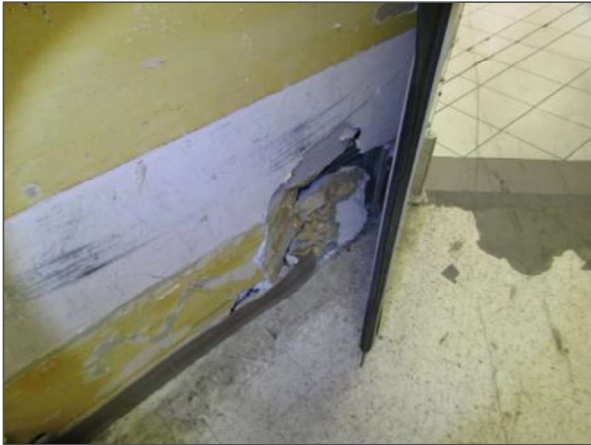
Damaged gypsum wall board was noted in multiple locations of the Site Building.
