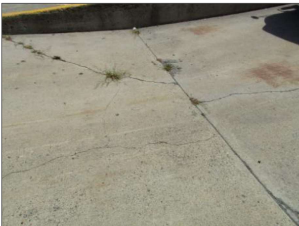
Localized areas of cracking were noted within the north concrete loading ramp.
