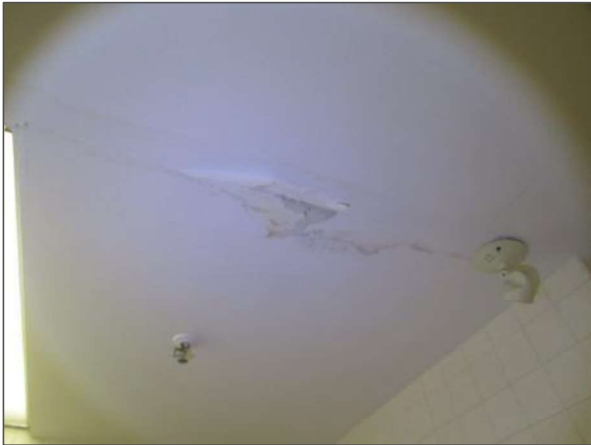
Moisture damage/stained gypsume ceiling board was noted in multiple locations of the Site Building.
