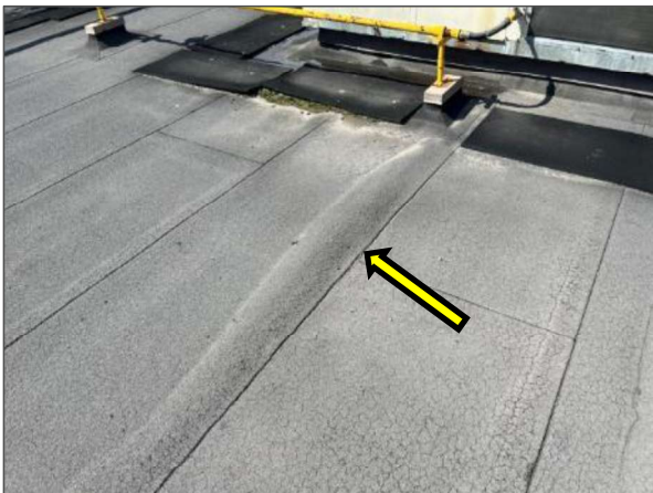
Areas of membrane blistering of the modified bitumen membrane roof system were noted atop Roof Section A5 in multiple locations.
