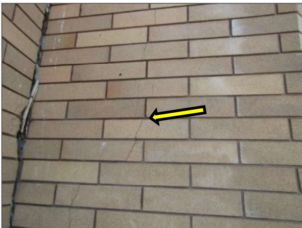
Localized areas of cracking within the brick veneer masonry were noted on the north elevation of the Site Building.
