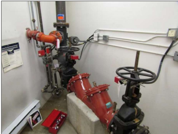
General view of a typical sprinkler riser and the observed backflow prevention device.
