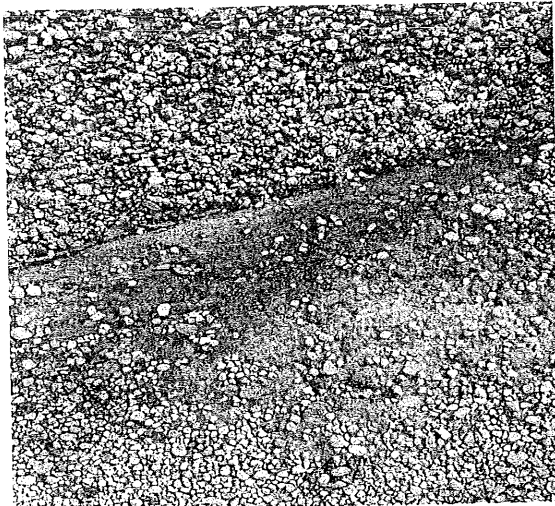
Localized tar paper exposure and likely roof leak
