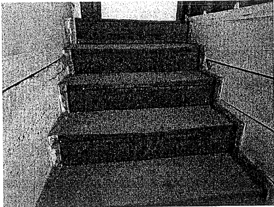
Uneven, unsafe stairway without handrailing
