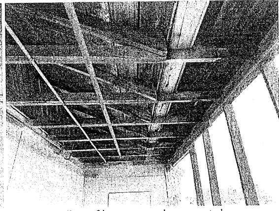
Rail side walk roof is not properly supported now.
