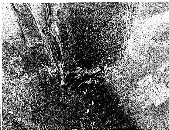
Heavy staining all CA room entry door frames
