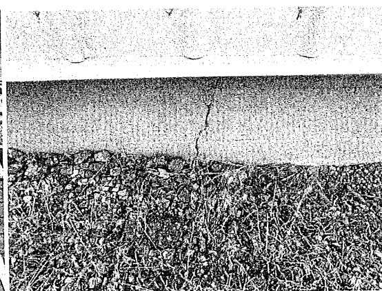
Open cracking in office building basement foundation
