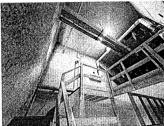
Non-standard guard openings and open structures
