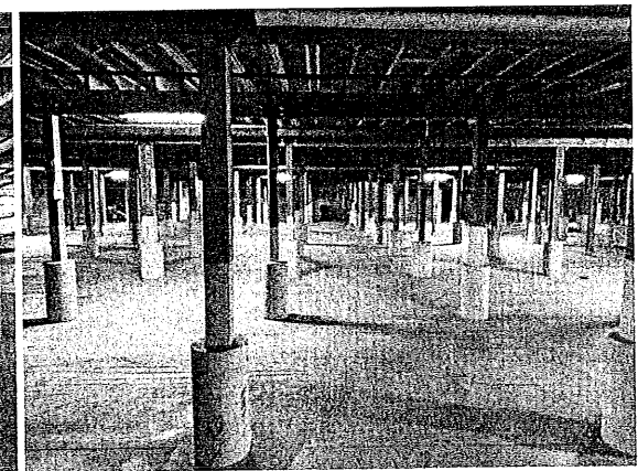
Warehouse and office basement post and beam structure
