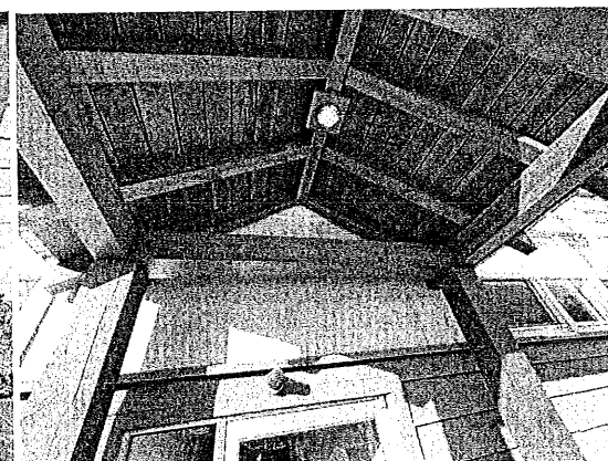
Wood structure not adequately secured to building
