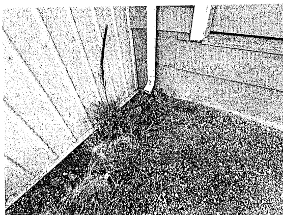
Roof runoff downpipes (RWL) require extension
